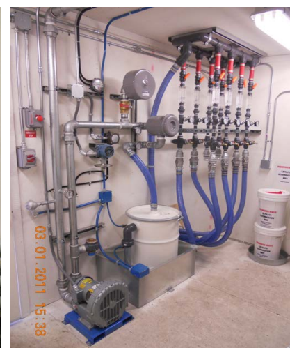
Figures 6-9. The soil vapor extraction and sub-slab depressurization systems installed at 314 Wendell Ave. are shown in these March 2011 photos. (Oasis Environmental Inc. photo, for DEC)
