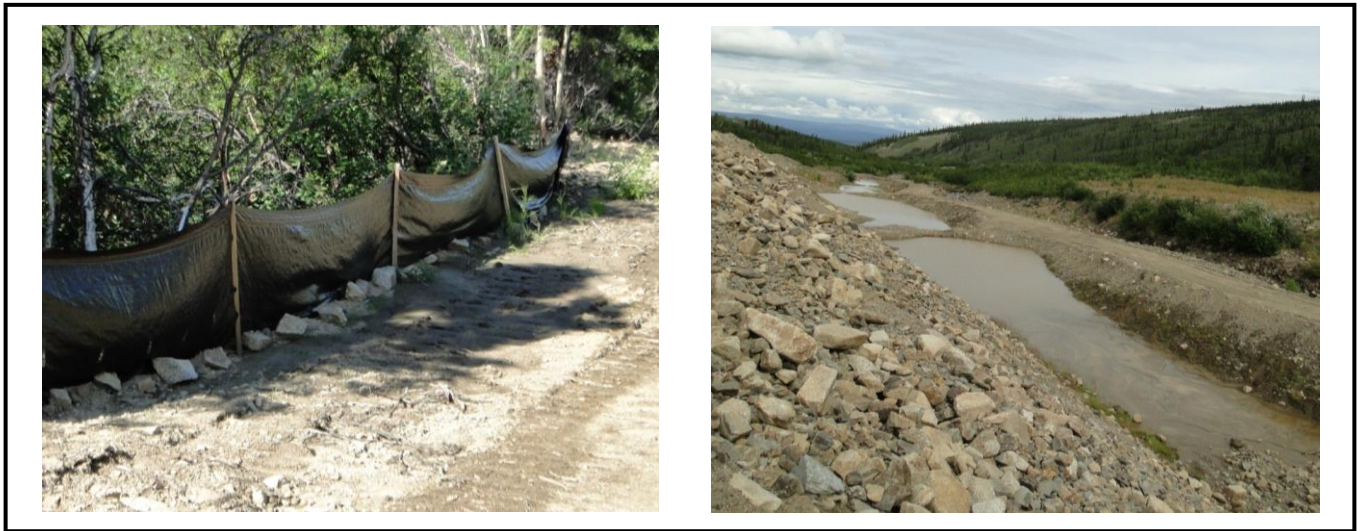
Examples of best management practices. Silt fence (left), elongated sediment ponds (right)
