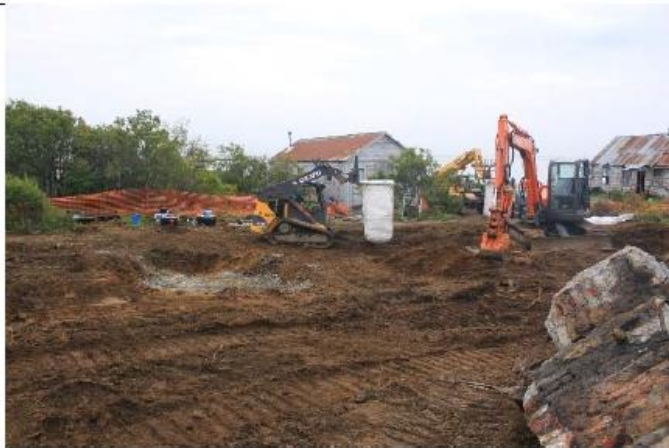
Power generation building site after demolition.
