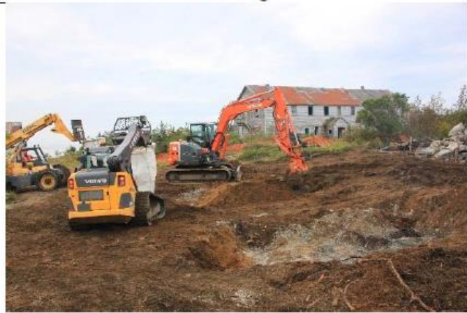
Beginning soil excavation at power generation building.
