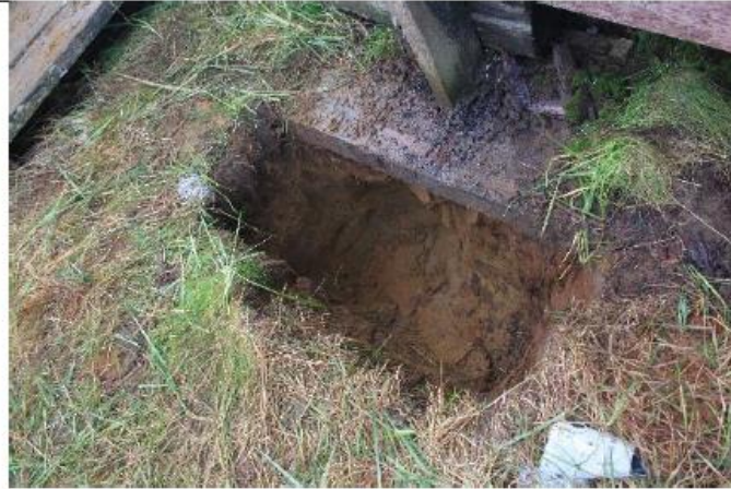
House Drum #1 excavation.
