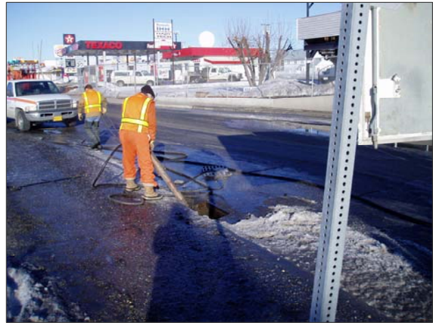
ADOT&PF personnel thawing stormwater system inlet during 2005 breakup
