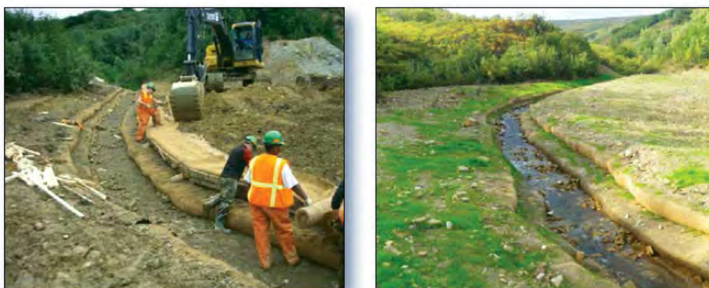
Figure 1-7. Slate Creek stream channel reconstruction (during construction: left, post construction: right [USEPA 2013]).
