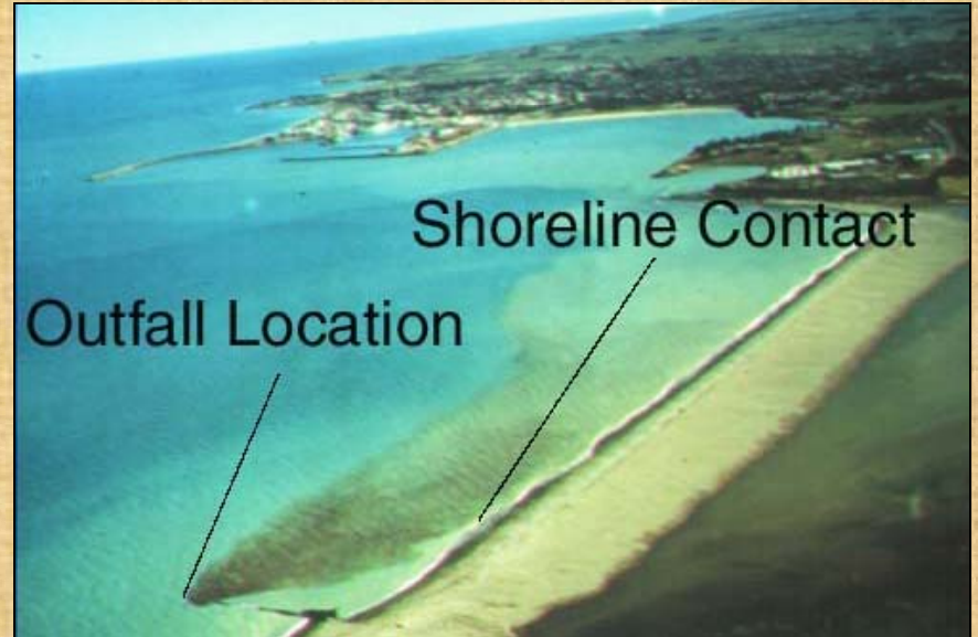
Wastewater outfall with boundary interaction
