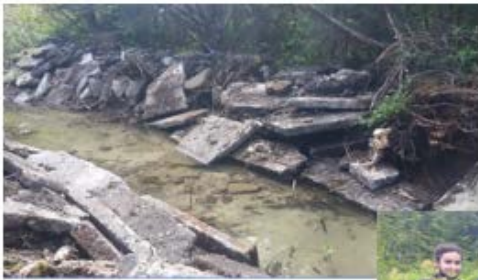
Debris removed from unnamed stream; a tributary of Odiak Pond.
