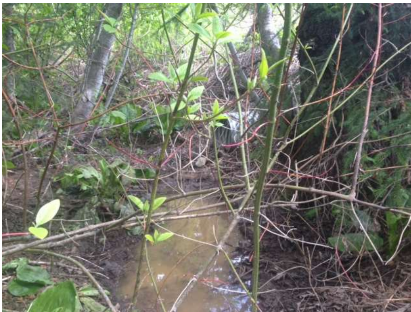
The Drainage ditch outlet after debris was removed. Photo: TWC Staff
