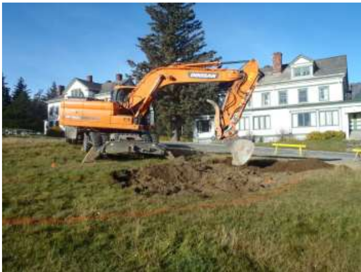
Installation of the bioswales. Photo: TWC staff
