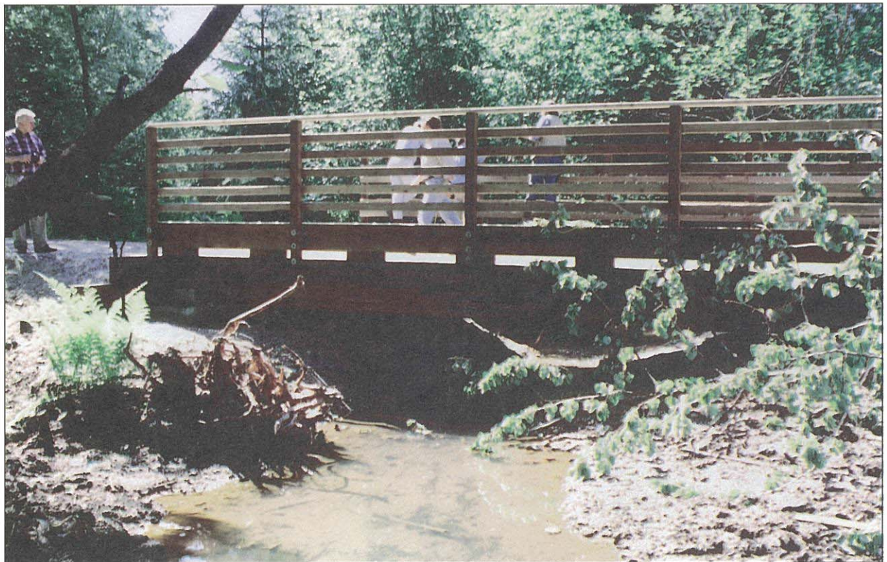
Figure 9.--Timber bridge used to replace a perched culvert on a private driveway. (Photo by NMFS).
