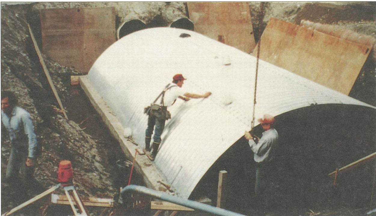
Figure 7.--Perched culverts being replaced with an arch culvert at Stephen-Richards Drive. (Photo by Jan Caulfield, CBJ).
