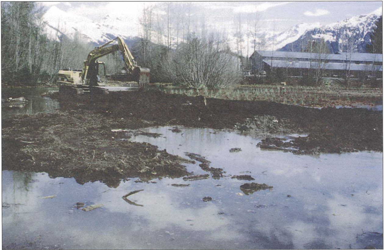
Figure 12.--The dredge pond that was developed into a stormwater treatment marsh. (Photo by NMFS).
