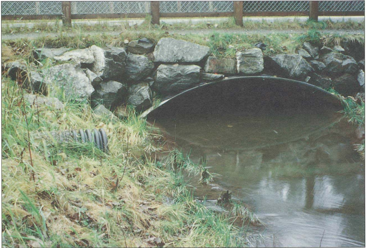
Figure 8.--Water flowing through new arch at Stephen-Richards Drive. (Photo by NMFS).
