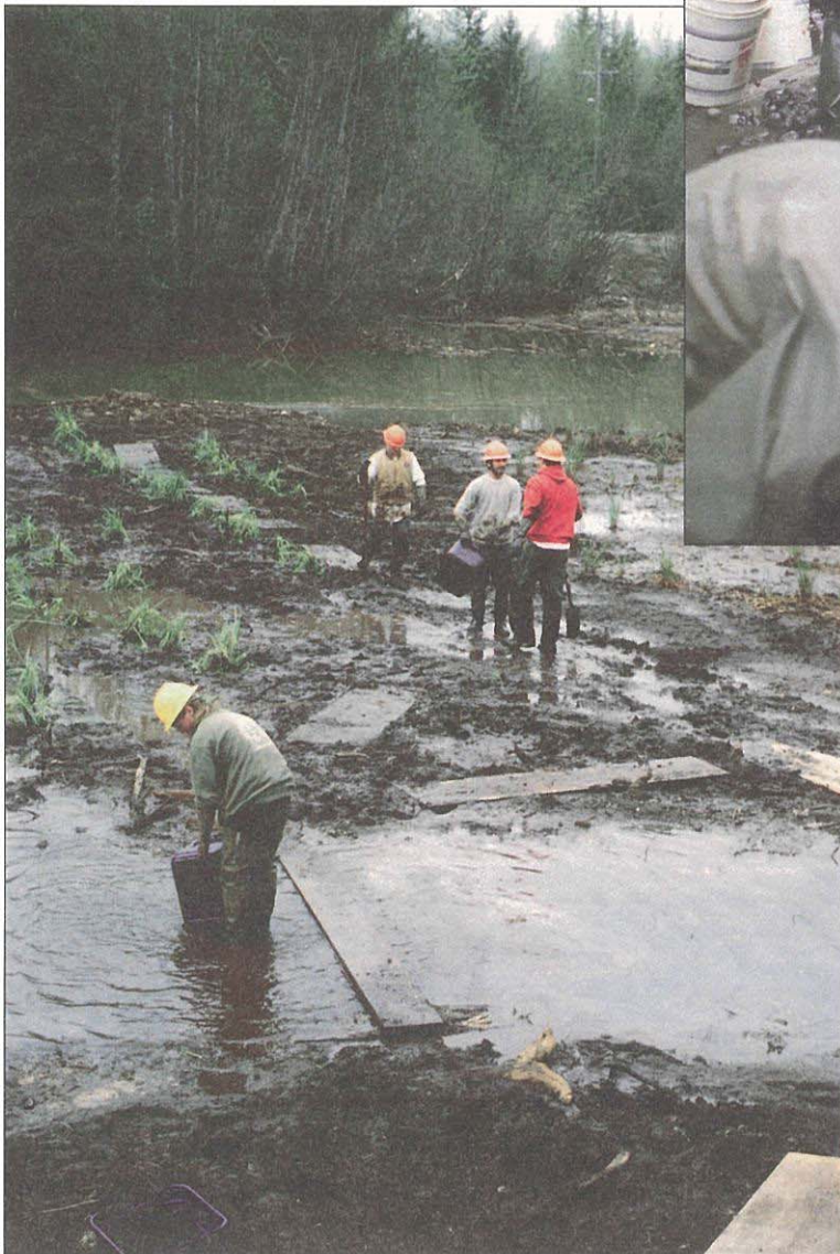
Figure 11.--Development of a stormwater treatment marsh in a dredge pond on the east fork of Duck Creek. (Photo by NMFS).
