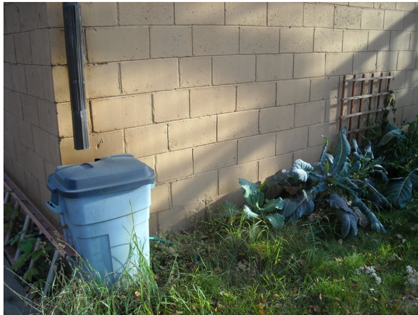
Figure 8. Additional water collection system installed to increase available water. Homeowner used a trash can with a hole cut into the lid.
