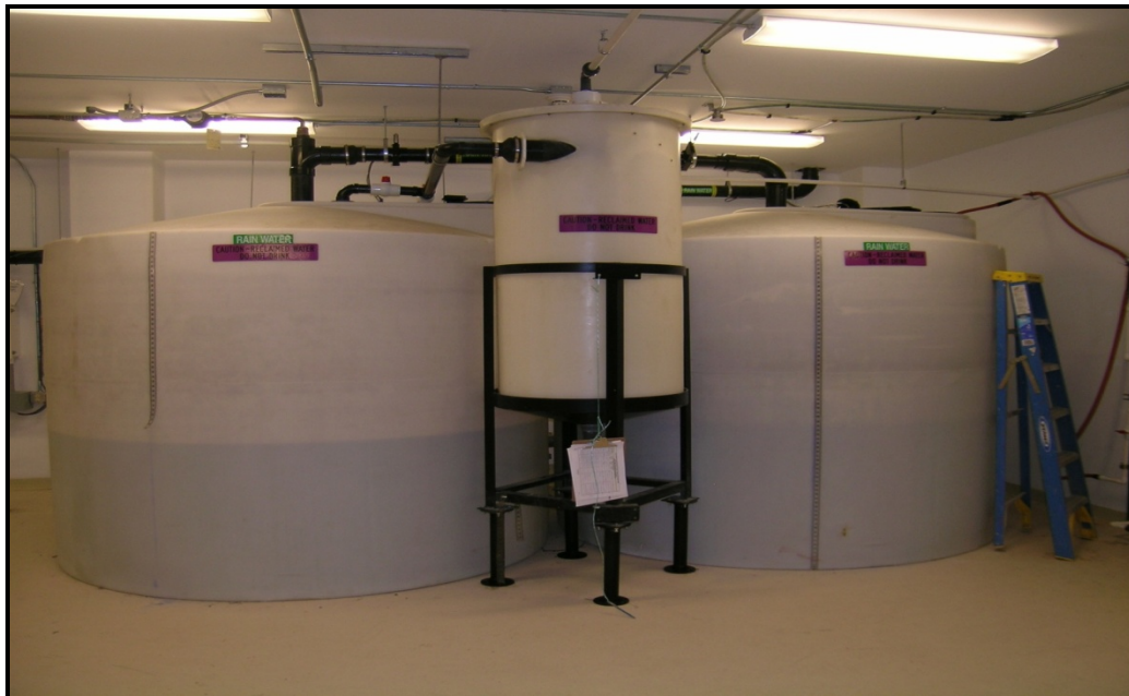
Figure 5. Two 1,500 gallon tanks are used to collect snowmelt and runoff, which are then used for gray-water applications, including toilets and outside faucets for watering rain-garden areas.
