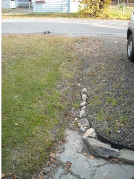
Figure 7. Remaining section of water diversion system that was previously used to help water get to the storm drain system.
