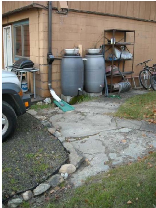
Figure 6. Rain barrels at backside of house, and water diversion set up that had previously been used to control flooding.
