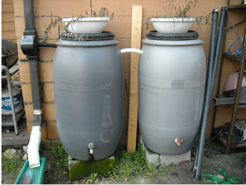
Figure 5. Photo of rain barrels at backside of house where water draining against house was an issue.
