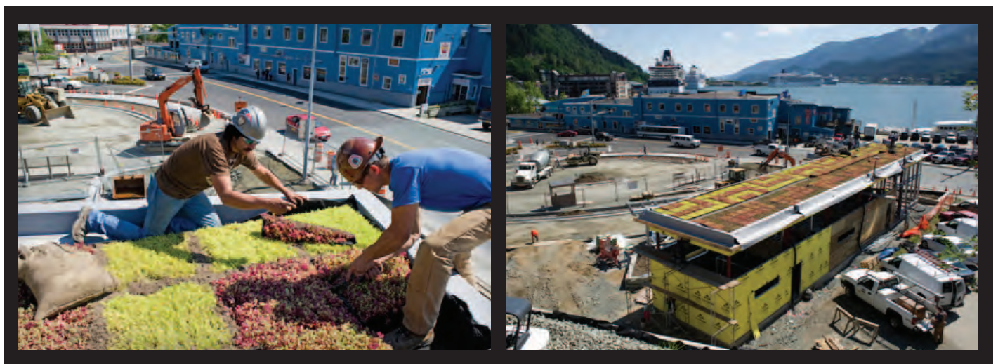
Figure Eight. Construction of a Green Roof on Juneau's Downtown Transportation Center. Juneau Empire, 2010.
