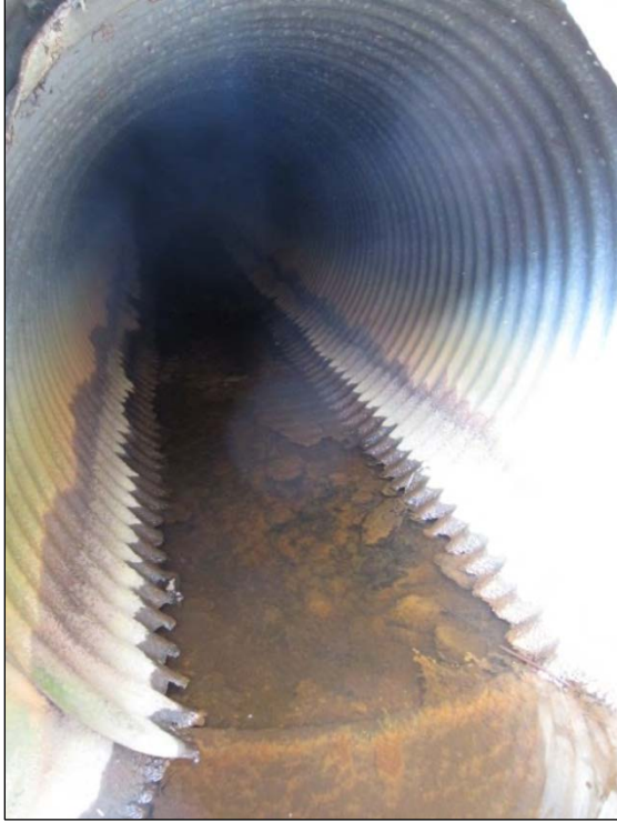
Figure E-19. Looking downstream at 42-inch CMP pipe inlet upstream of Lake Street.
