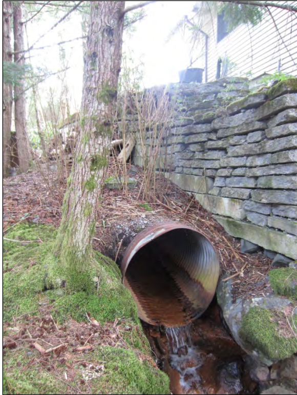
Figure E-21. Looking east (upstream) at the 42-inch CMP outlet on private property west of Lake Street.
