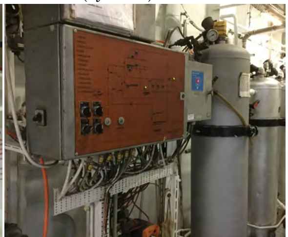
Photo 59: MarineFloc OWS Control panel
