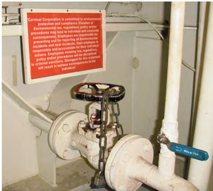
Photo 16: Closed discharge valve
