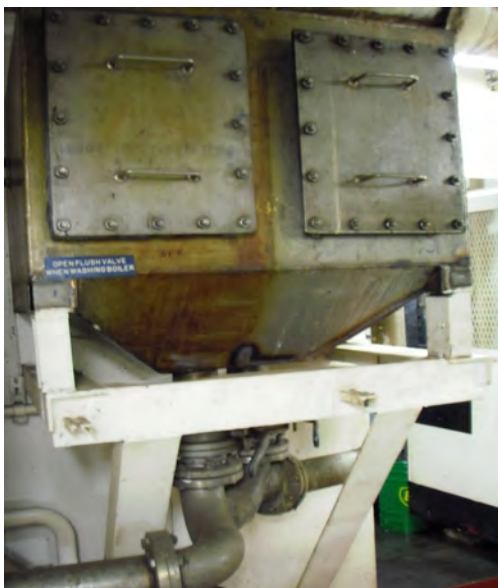
Photo 7: Boiler drain, soot trap
