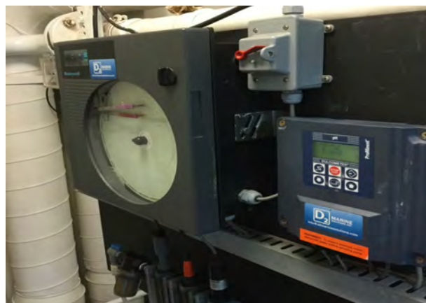
Photo 50: Chart Recorder for pH & Chlorination
