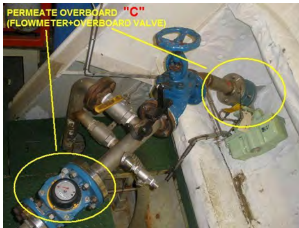
Photo 12: Overboard valve, flow meter, and Sample port
