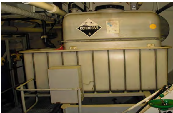
Photo 28: Chemicals, properly stored in containment basin
