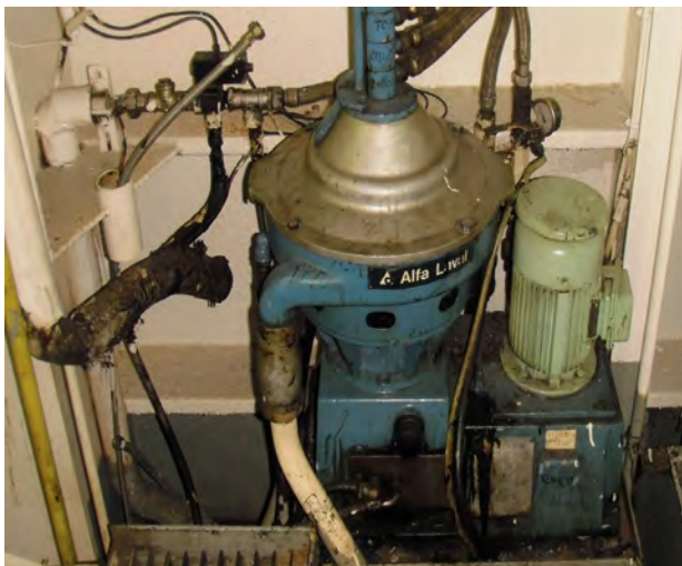
Photo 56: OWS separator (dynamic)
