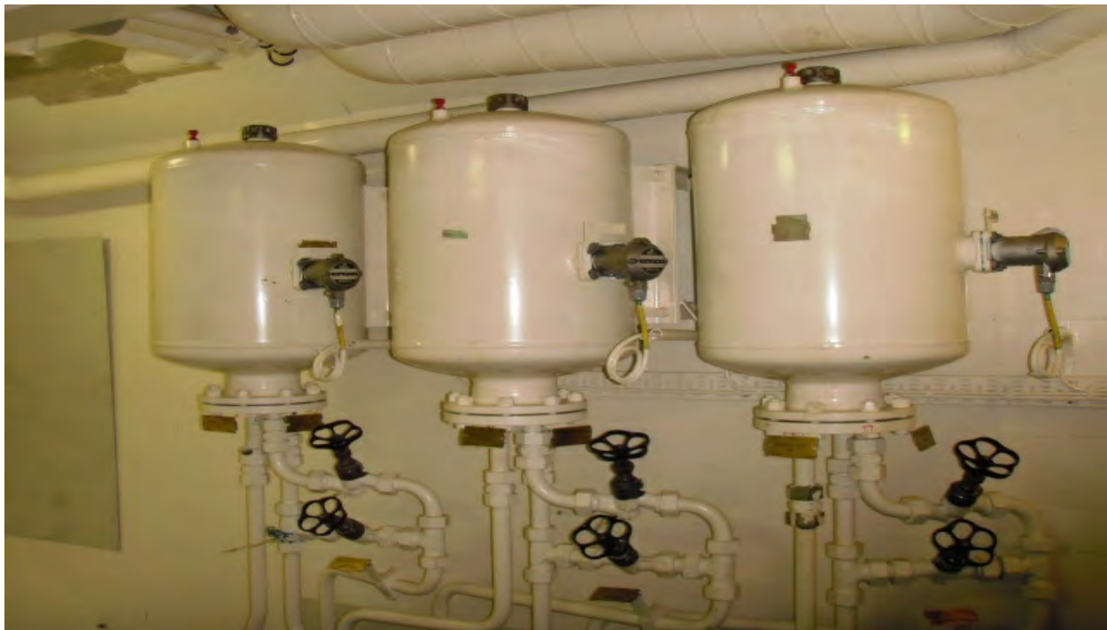
Photo 60: Oil to Sea gravity tanks
