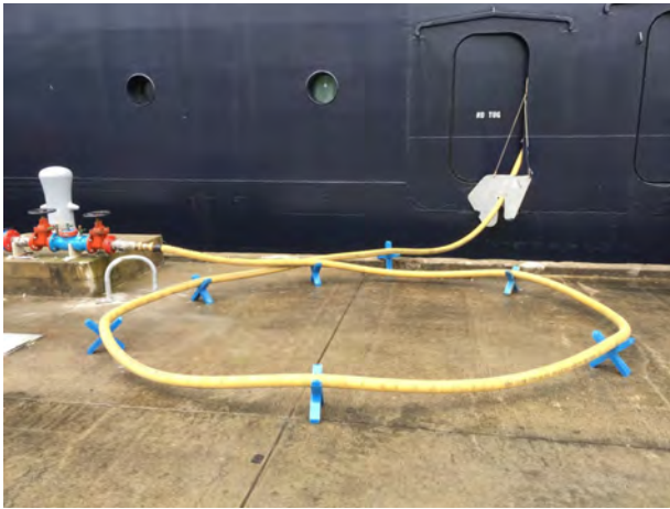
Photo 47: Elevated Potable water hose
