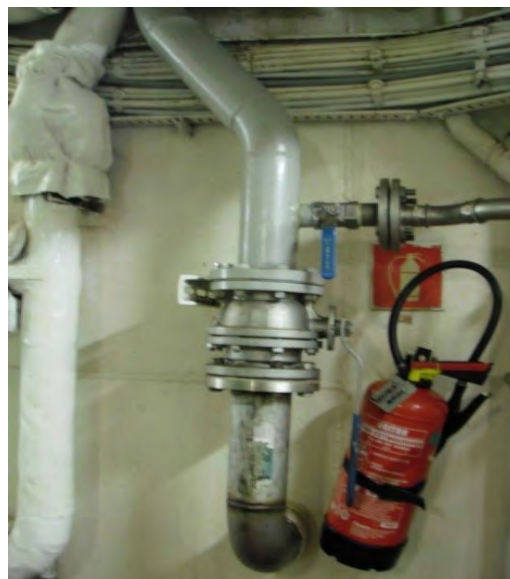
Photo 8: Boiler drain line
