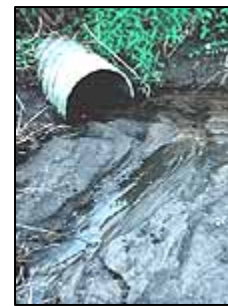
Stormwater outfall/discharge
