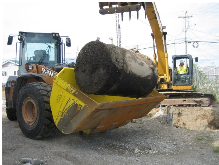
Underground Storage Tank Removal next to the Ferguson building.
