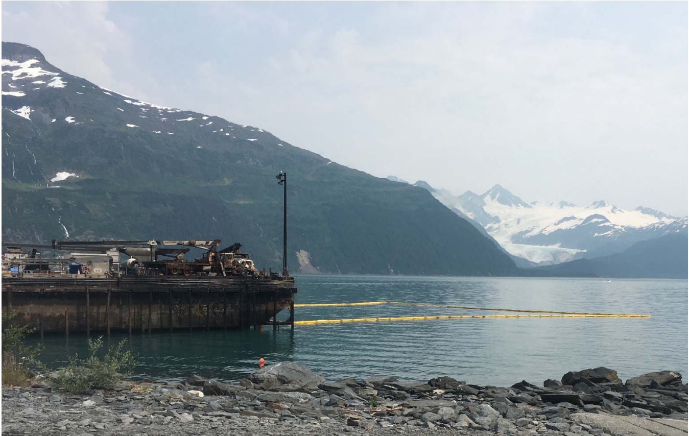
Alaska Chadux Corporation deployed containment boom around barge location. ADEC 7-9-19
