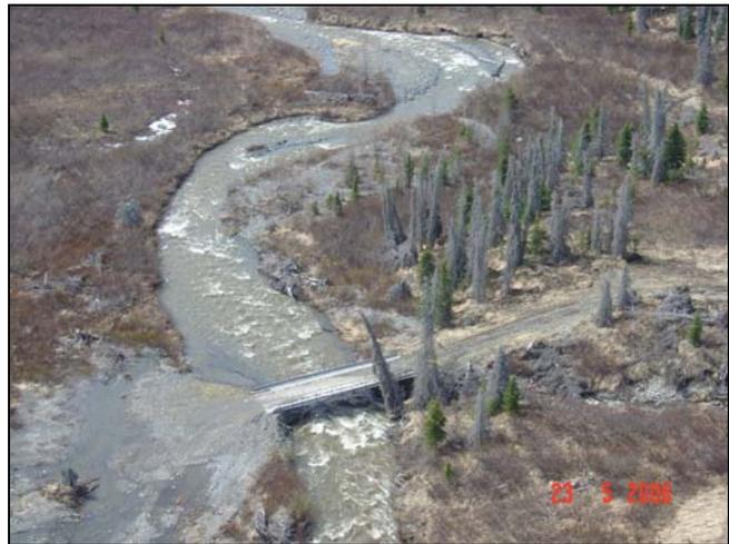
The bridge across the Water Hole Trail reduces direct impacts from ATV crossings the stream, yet high water flows in the spring are eroding the gravel around the bridge, threatening the long-term stability of the bridge.
