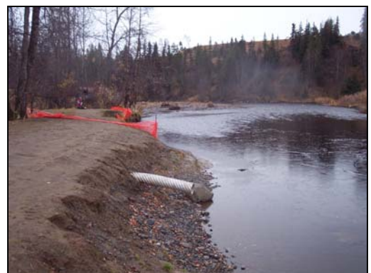
In the photo series above, the Picnic Hole erosion over a two year period is evident (May 2004, May 2005, October 2006, respectively).
