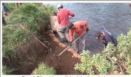
Backfill with soil behind coir log
