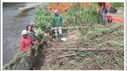
Install spruce tree revetment
