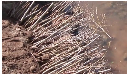
Cut willows leaving about 8 inches exposed
