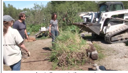
Install vegetation mat
