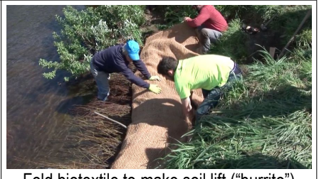
Fold biotextile to make soil lift ("burrito")
