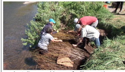
Install second layer of willow cuttings
