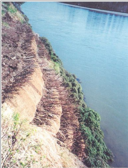
BRUSH-LAYERING with cabled spruce trees to protect toe
