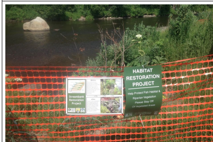
Install fencing and signage
