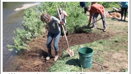
Water and compact backfill over willows
