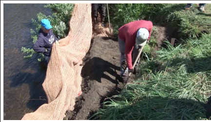
Lay down biotextile and backfill with gravel
