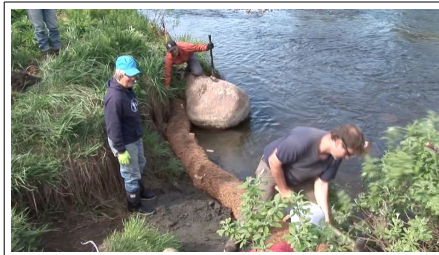
Install coir log
