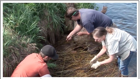
Install first layer of willow cuttings
