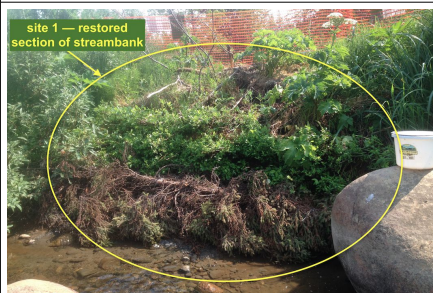
Site 1 on July 6, 1 month after installation
