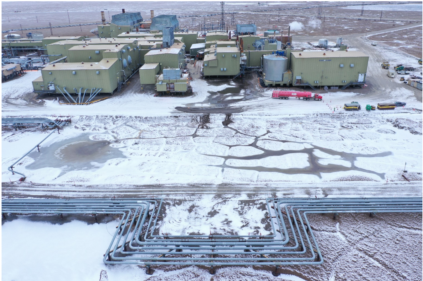
Image collected during an UAV overflight on 10/21/2019, showing the affected area (dark colored fluids on gravel pad and within tundra polygonal troughs). Image collected by ACS and provided by APSC.
