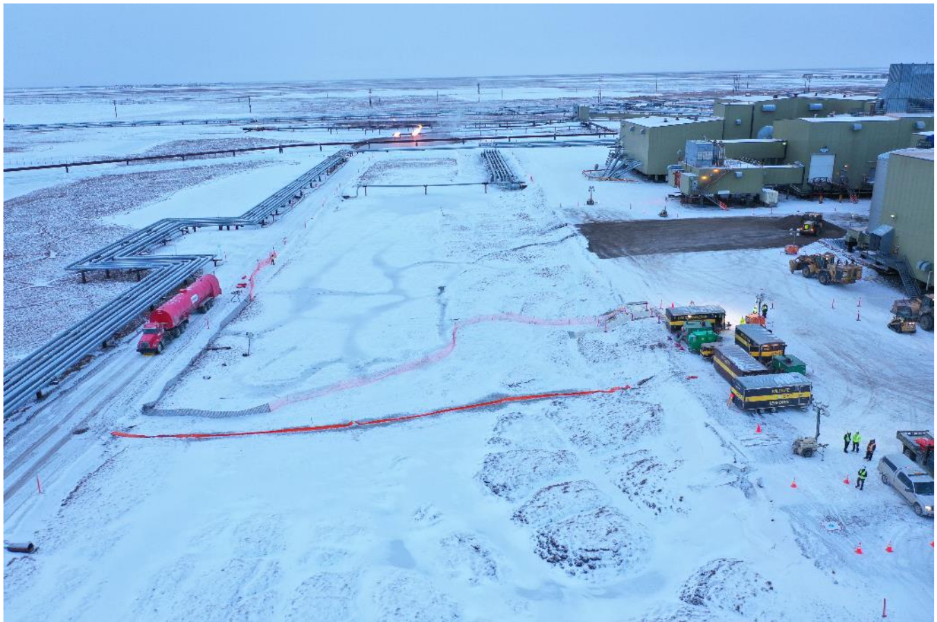
Image collected during an UAV overflight on October 22, 2019, before off pad flush and recovery tactics were initiated but after wildlife fencing had been put up, containment boom deployed, and gravel removal conducted. Image collected by ACS and provided by APSC.
