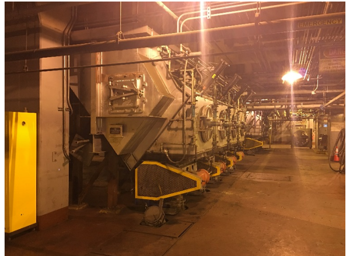
Bottom Ash collection point from boilers
