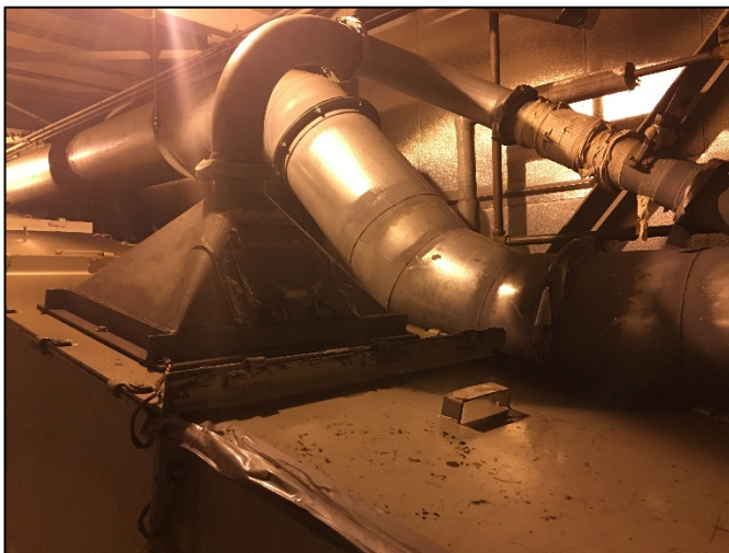
Coal Dust Collection Vacuum Suction on Level 6
