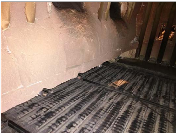
Forged nozzles shown with air flow parallel to the grate. No pipe nipples were used for Boilers 4, 6, 7, and 8.
