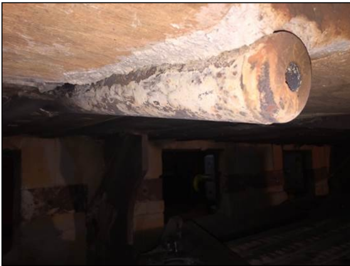
Forged 3/4" aperture nozzle welded into 2" pipe for front wall.
