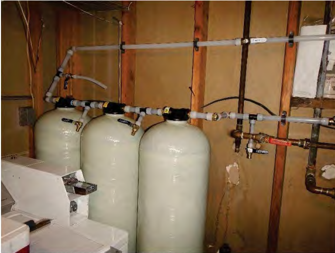
Photo 1: We collected a post-treatment sample (407429-D) from the granular activated carbon (GAC) treatment system outlet at 3350 Holden Road. (December 14, 2016)
