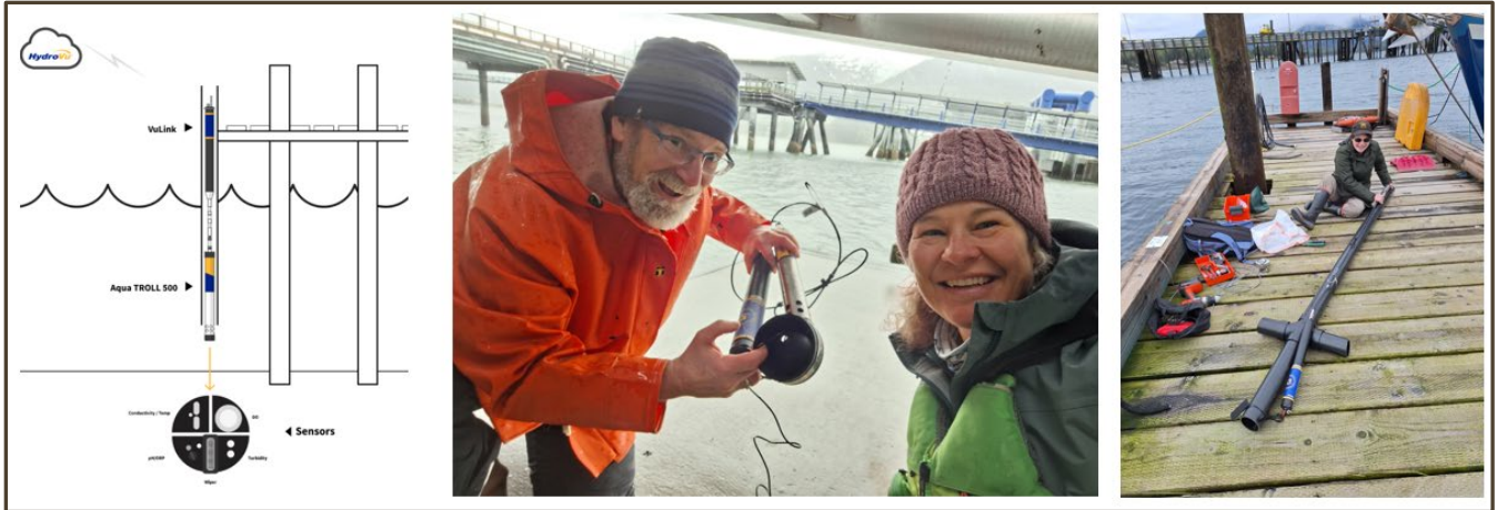
Figure 8. A schematic of water quality sensors equipped with HydroVu (left), sensor installation (middle in Juneau, right in Ketchikan).
