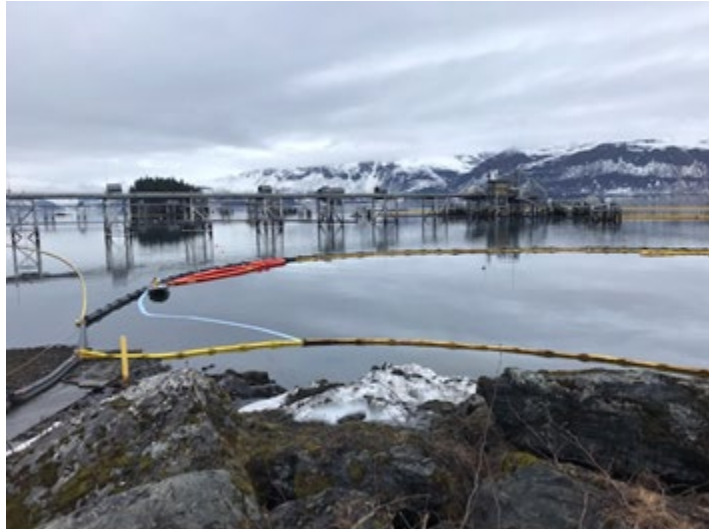
Figure 1. Containment boom looking west at the VMT on April 21, 2020. Courtesy ADEC
