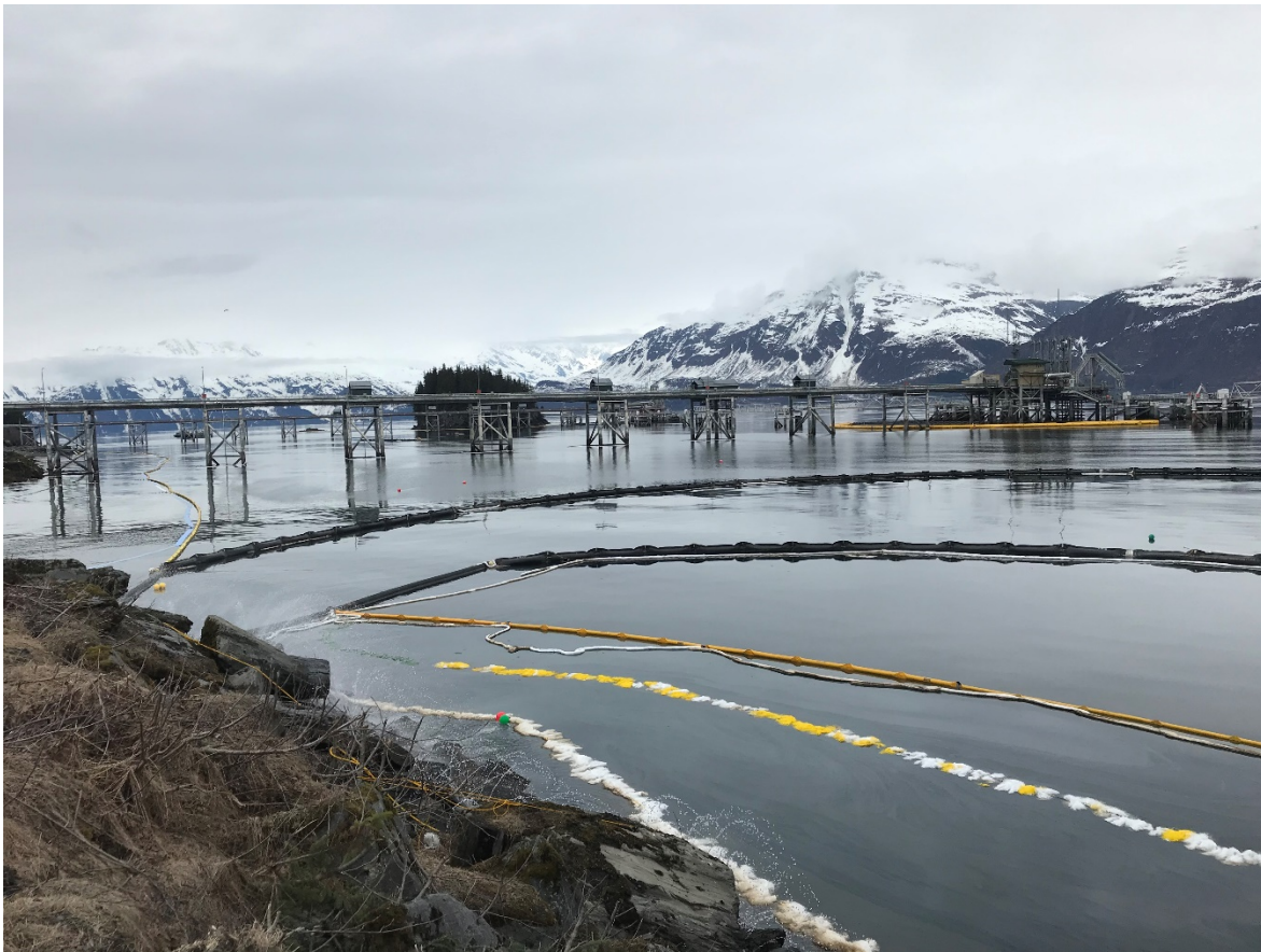
Figure 1. Containment boom looking west at the VMT on May 1, 2020 . Courtesy ADEC
