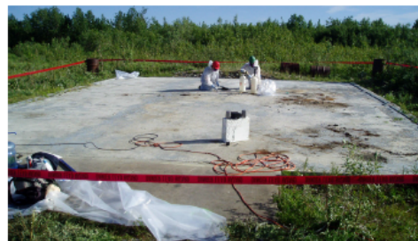
Lead paint is removed from concrete prior to demolition at a site in King Salmon, Alaska
