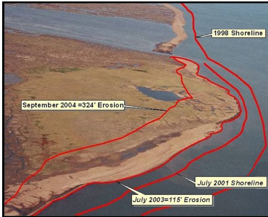
2 3 J.W. Dalton Drill Site Erosion. Located east of Utqiagvik on the Beaufort Sea near Teshekpuk Lake and Point Lonely DEW line site. 4 This photograph was taken in 2003; between the summers of 2003 and 2004 over 300 feet of shoreline eroded away along part 5 of the site. Approximately 600 feet of coastal plain were lost over a 6-year period. Photo provided by BLM
