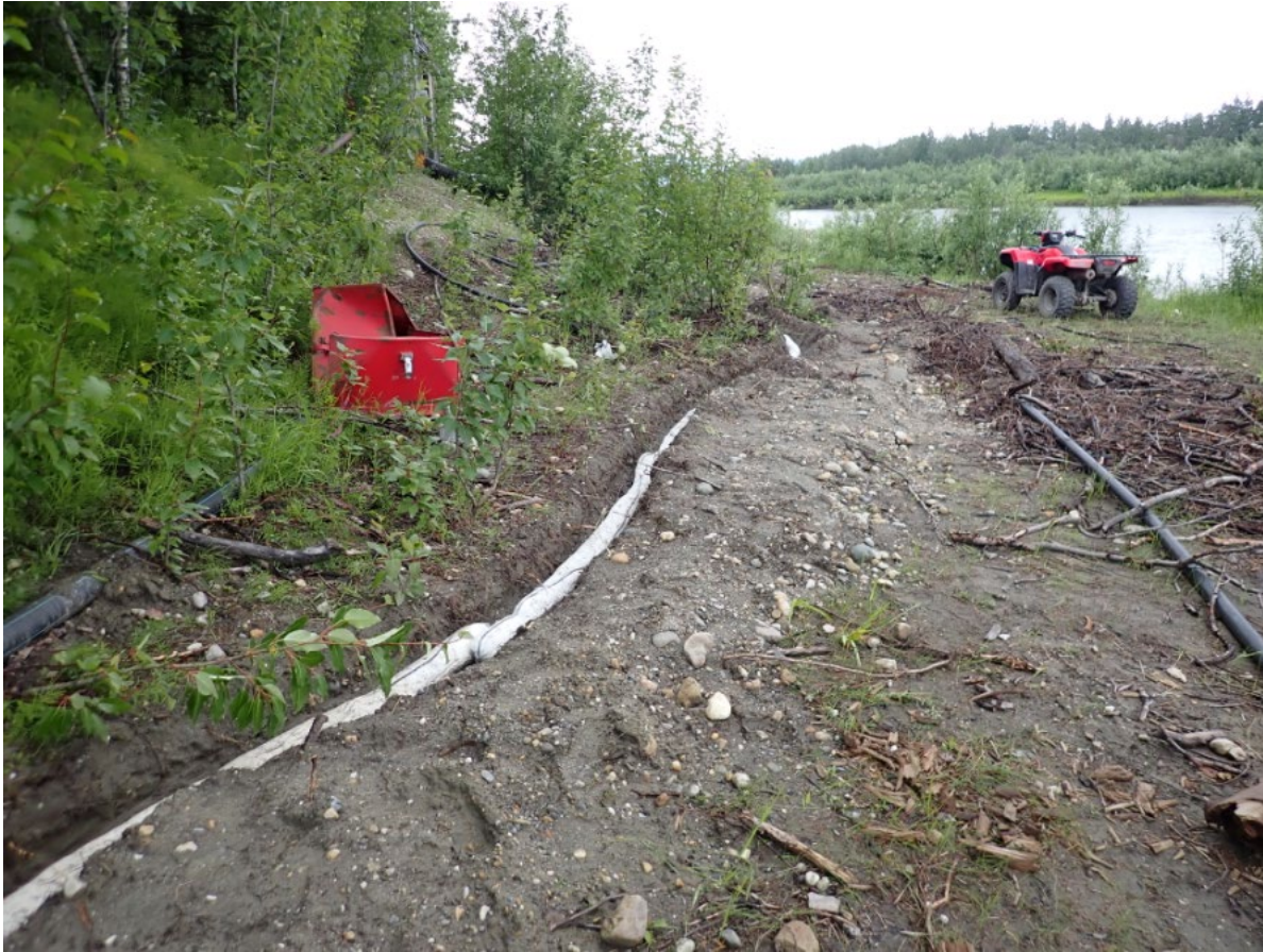
Sorbent boom in a trench along the riverbank to prevent the spill from reaching the Kobuk River, Shungnak, Alaska (Photo: J. Miller/ADEC, June 29, 2020)
