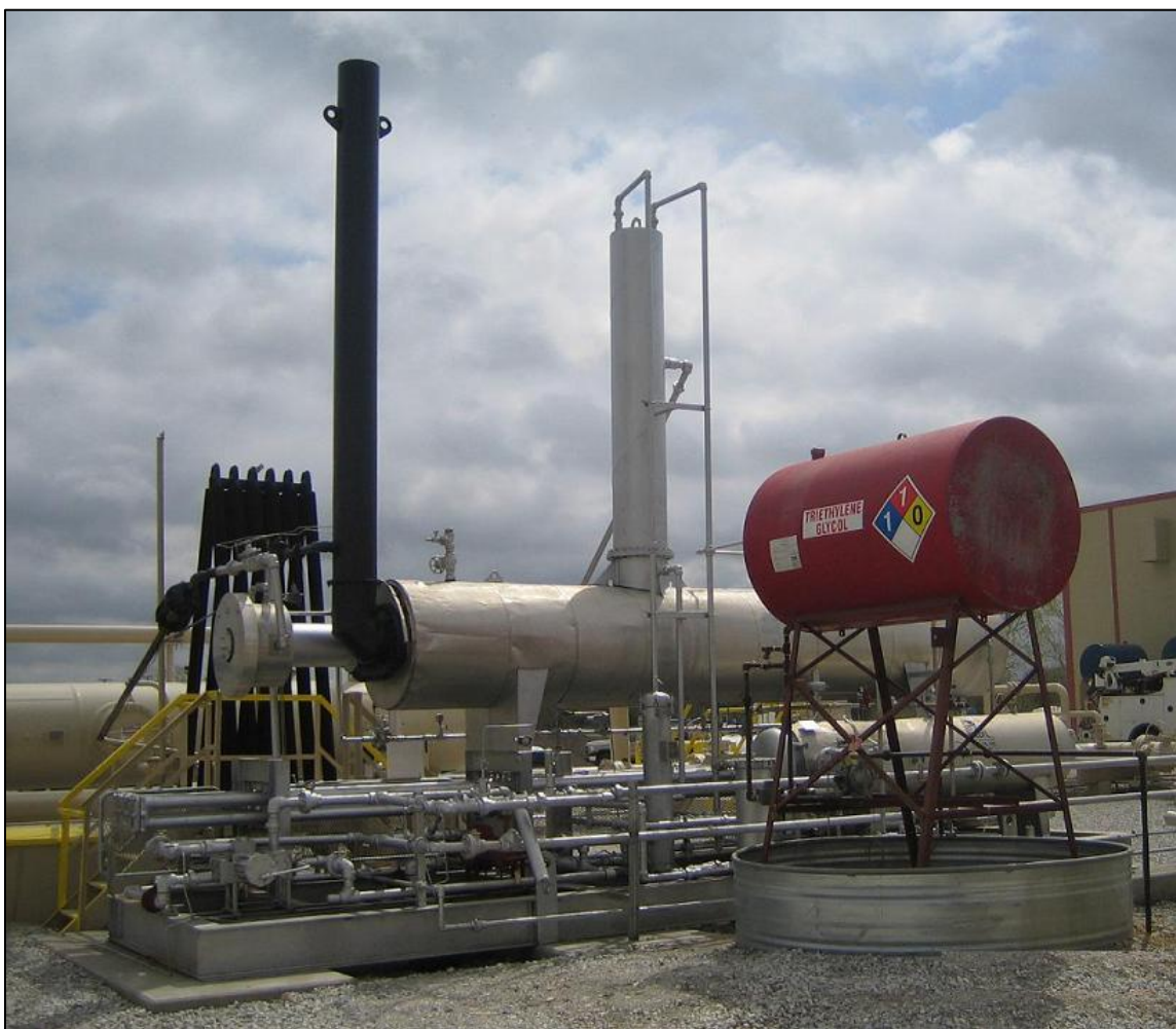
Figure 3-5. Dehydrator
