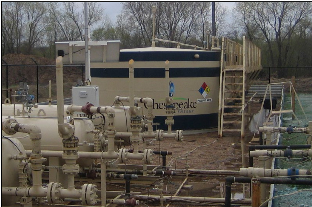
Figure 3-15. Produced Water Tanks
