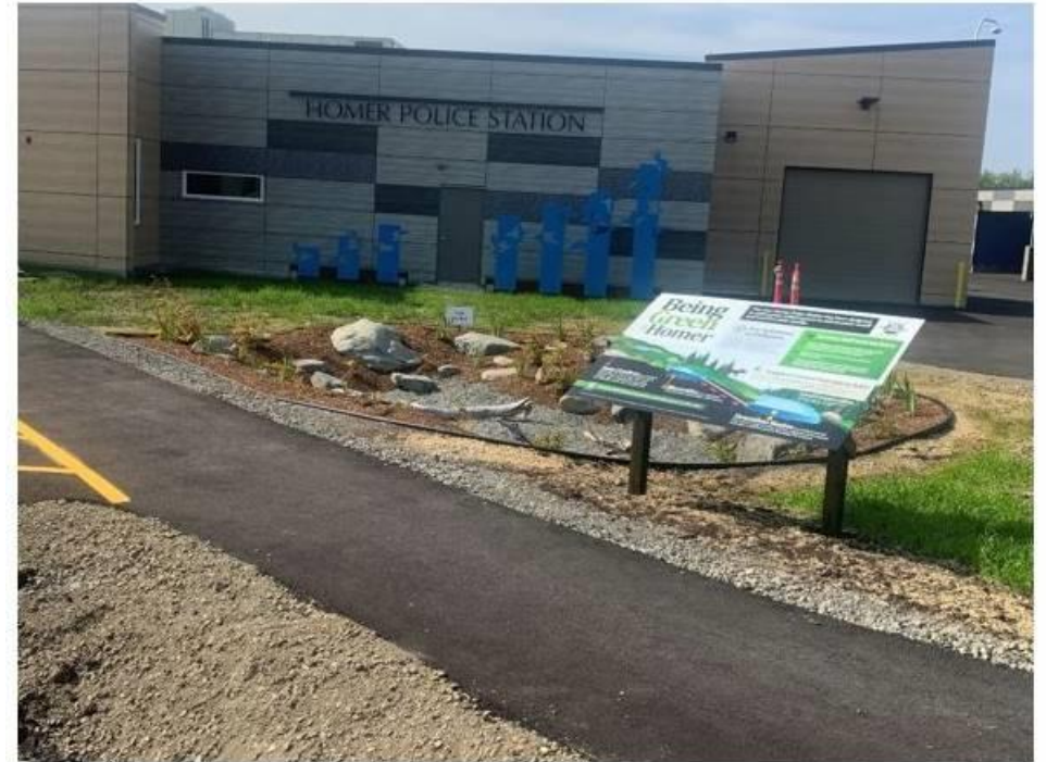
New RAIN GARDEN - site drainage directed to garden to slow peak storm water and filter sediments
