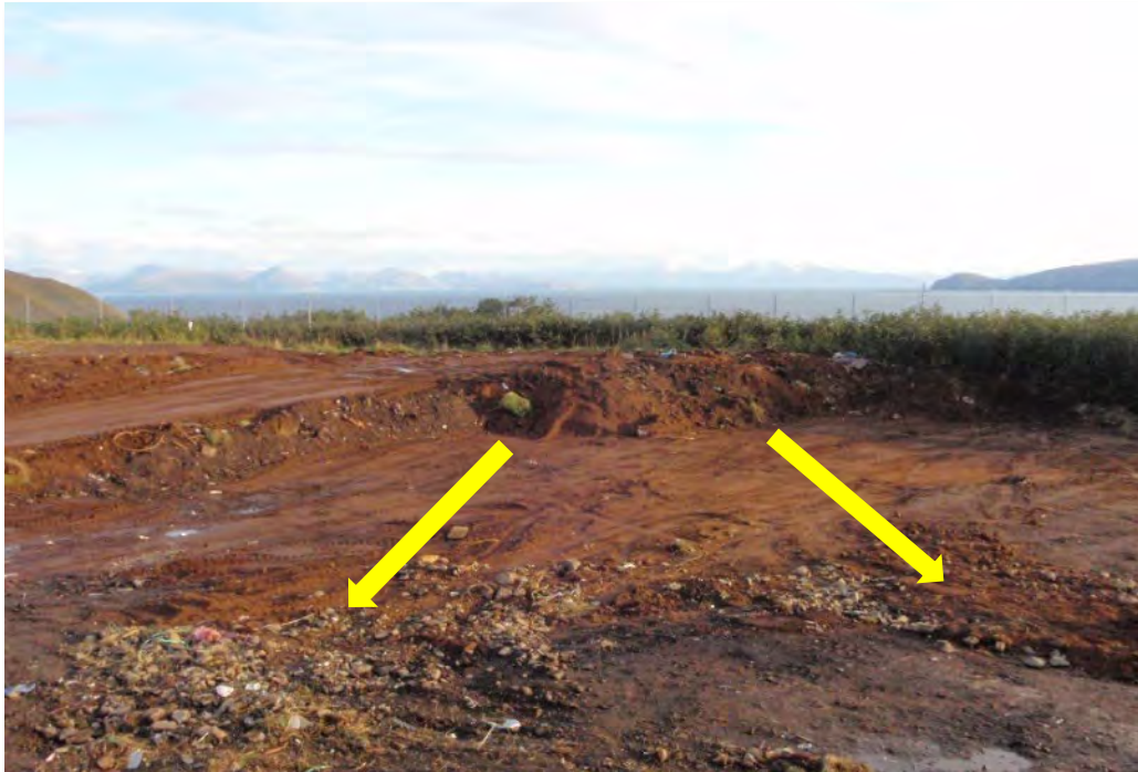
Cover material at the working face graded to promote water drainage away from the waste. Water is draining away from the working face following the arrows.
