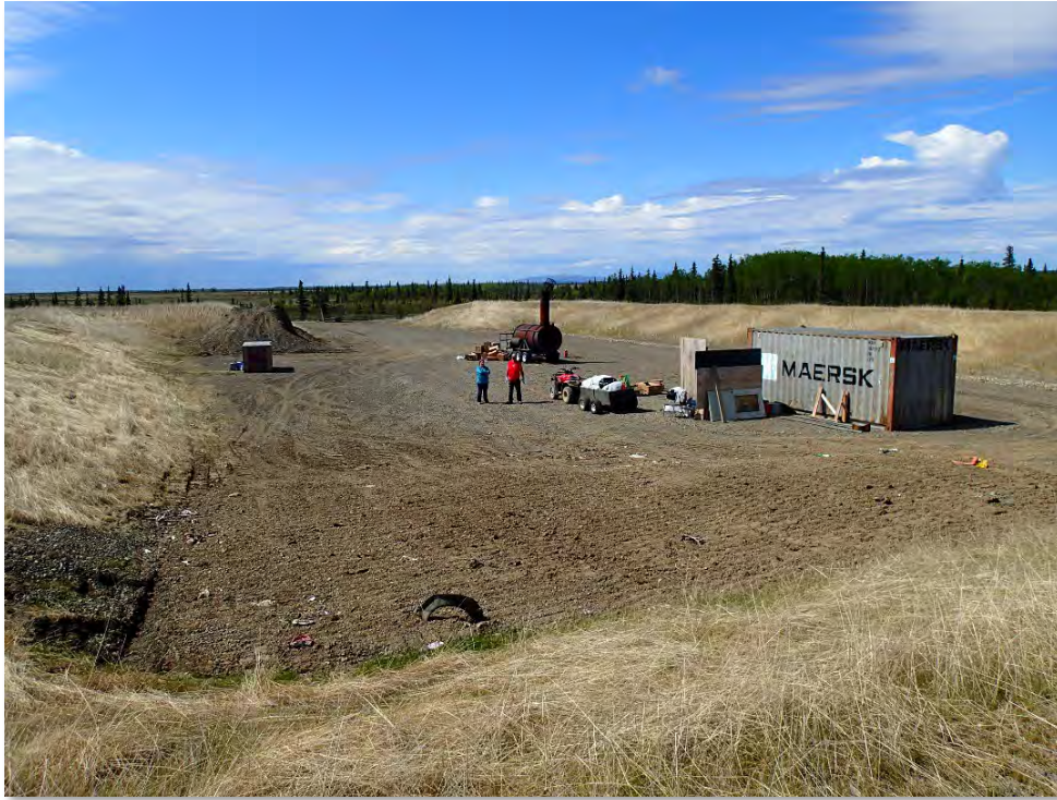
Well-managed landfill that is not likely to attract wildlife.
