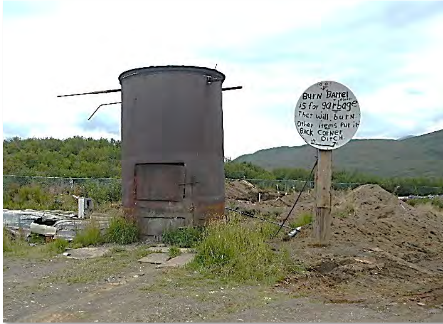
Burn unit with a sign nearby describing where burnable and non-burnable waste should be placed.
