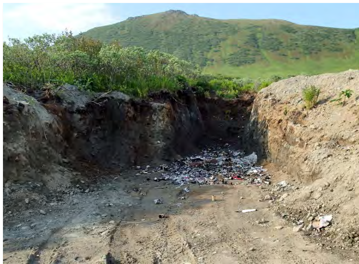
Working face at a trench-and-fill landfill.
