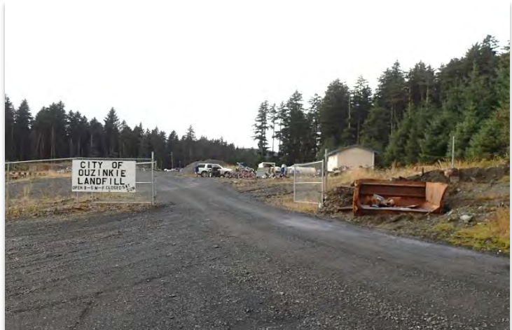
Landfill with drop off bin for waste outside of the gate.
