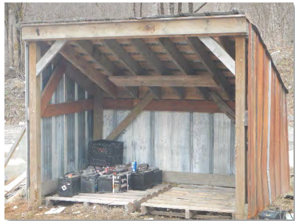
Covered storage shed for lead acid batteries.
