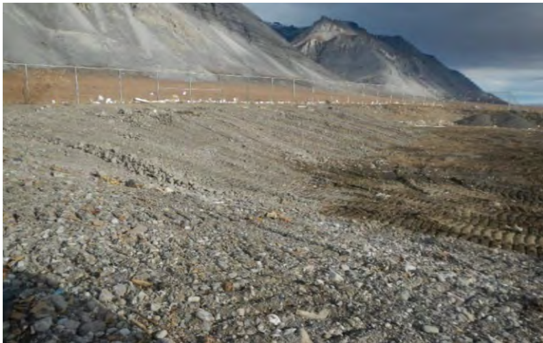
Working face that has been compacted and covered.
