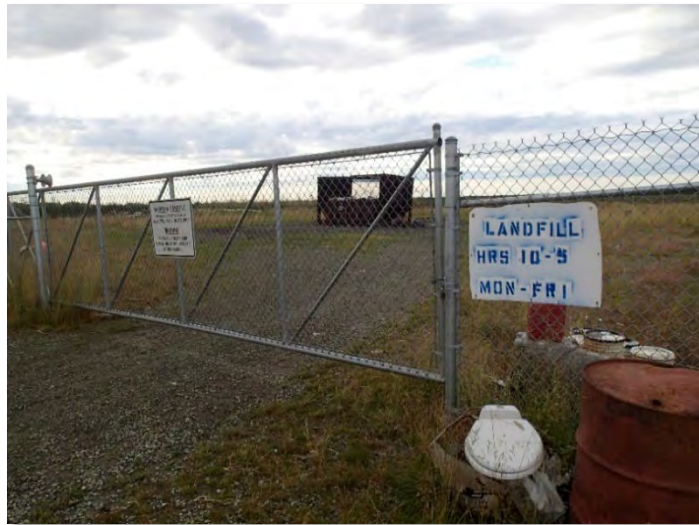
Locked landfill gate with open hours listed.
