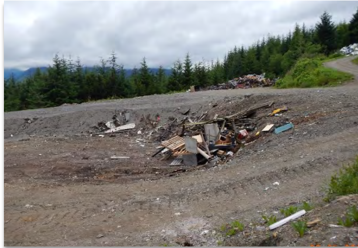
Working face at an area fill.
