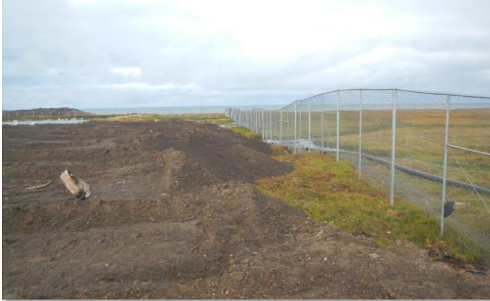
Waste recently covered.
