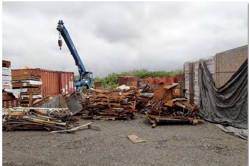
C&D debris staged for backhaul in the community.
