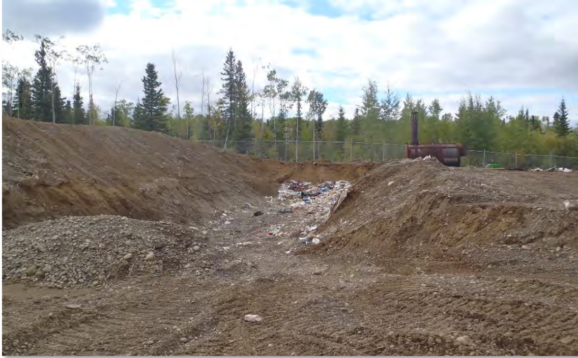
Trench-and-fill working face.
