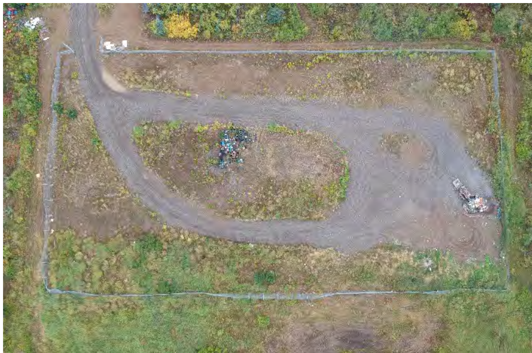
Well-maintained road within the landfill.
