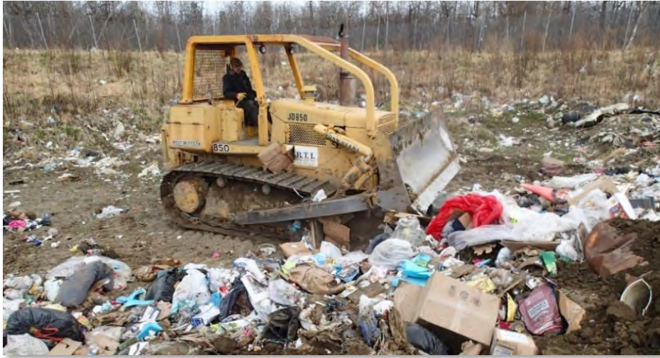
Operator using a dozer to consolidate waste.
