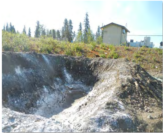
Septage trench with lime added.
