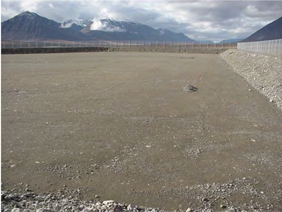
An example of a landfill built on a pad above permafrost prior to waste placement
