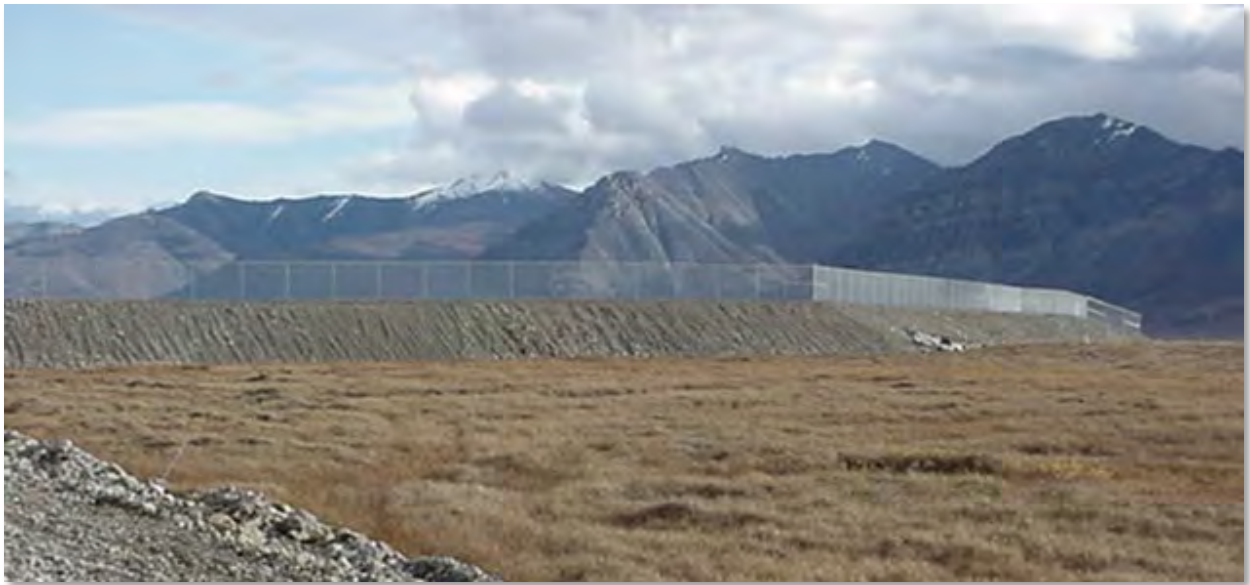
Landfill built on a thick pad to protect the permafrost beneath it.
