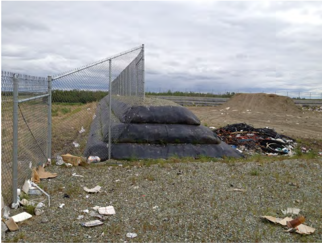
Berms and fencing surrounding an above-grade area fill in wetlands. The berms provide a wall against which to compact waste and help keep the landfill separate from the wetlands, while the fencing helps to contain windblown litter.
