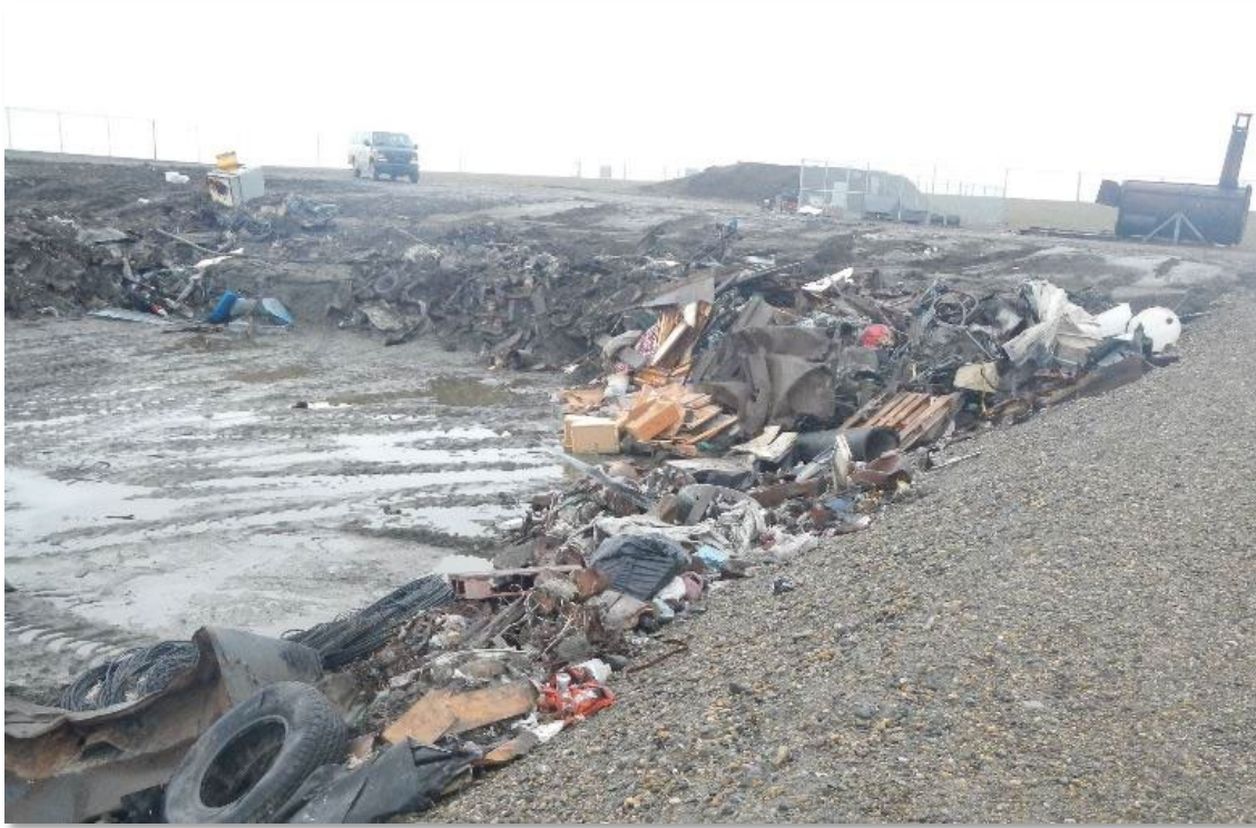
Working face at an area fill landfill.
