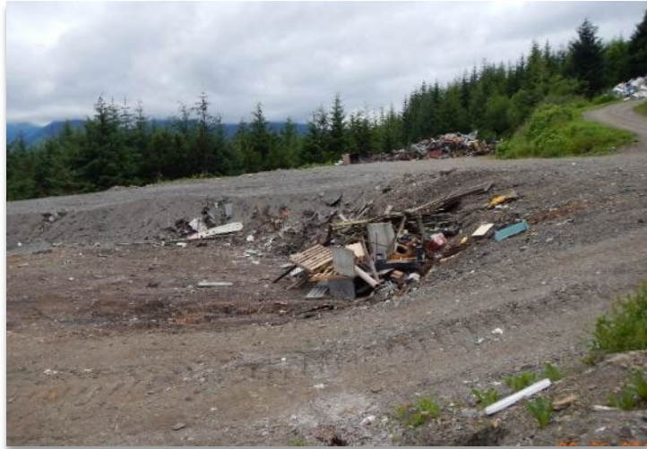
Working face at an area fill.
