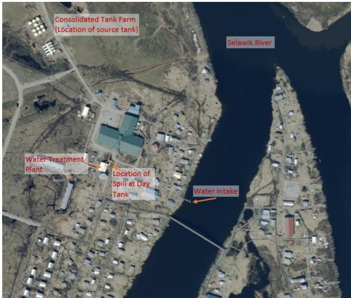
City of Selawik and Location of Spill (Image credit: Google Earth)
