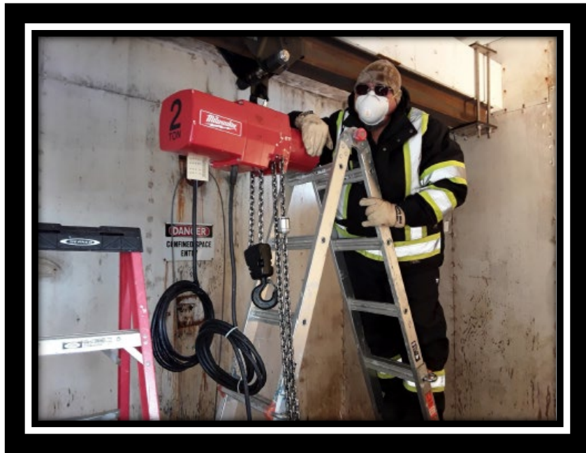
NSHC RMW, Richard Kuzuguk, assisting with the installation of an electric chain hoist
