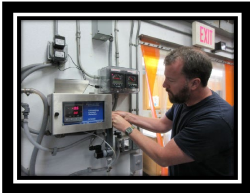
RMW Theo Graber inspecting the Streaming Current Detector in Nanwalek
