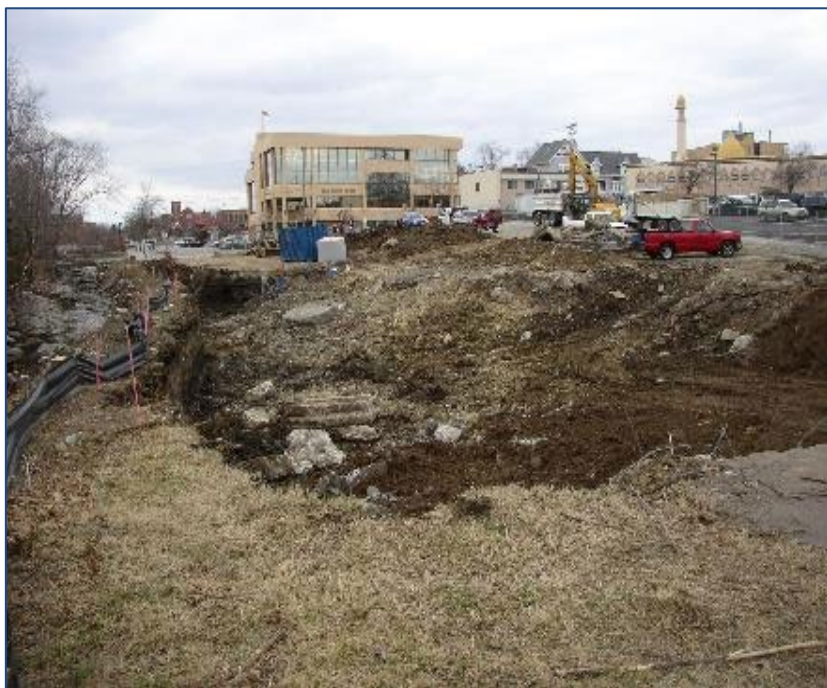
Before: Former bulk oil facility
