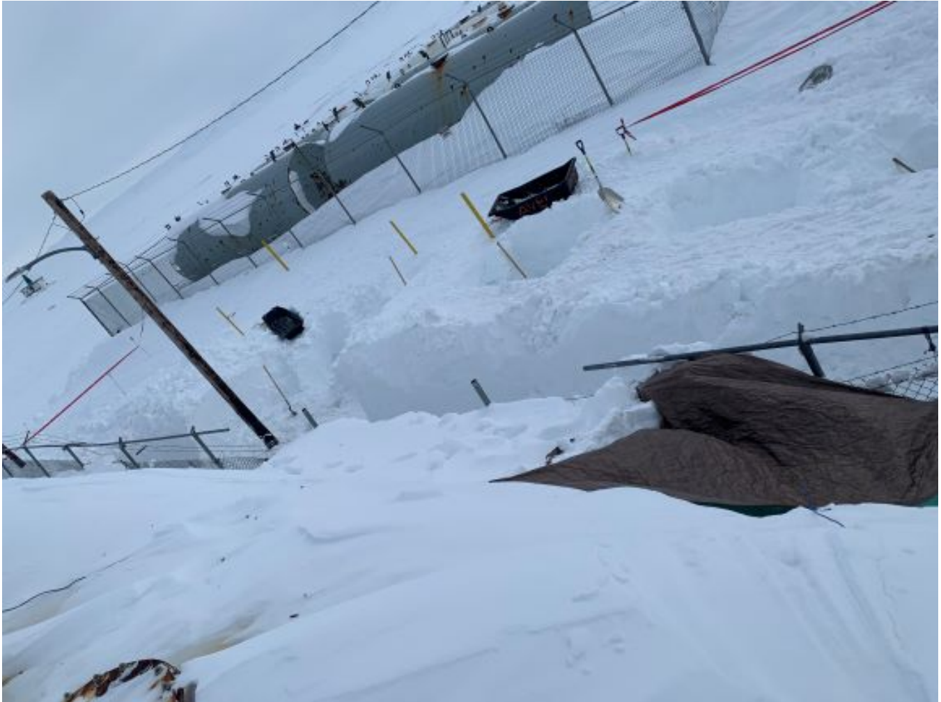
Photo 1. Survey holes to check for additional contamination outside of secondary containment. (Photo provided by Scott Stiker, March 3, 2021)
