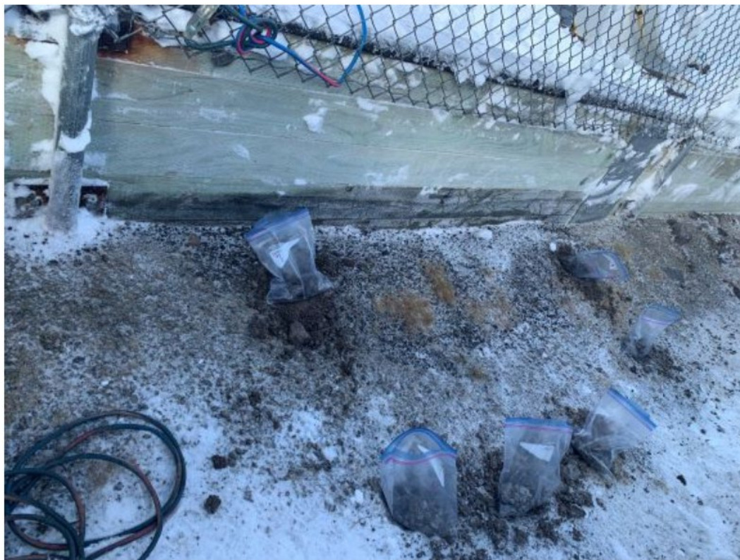
Photo 2. Soil samples collected on the east wall where diesel was found outside of secondary containment. (Photo provided by Scott Stiker, March 18, 2021)
