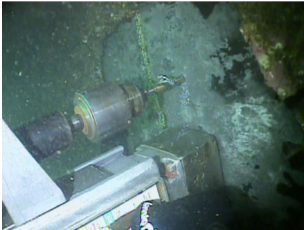
(Photo Credit: Global Diving and Salvage: Diver using a magnetic drill press to open an exploratory hole in the hull – 8/20)
