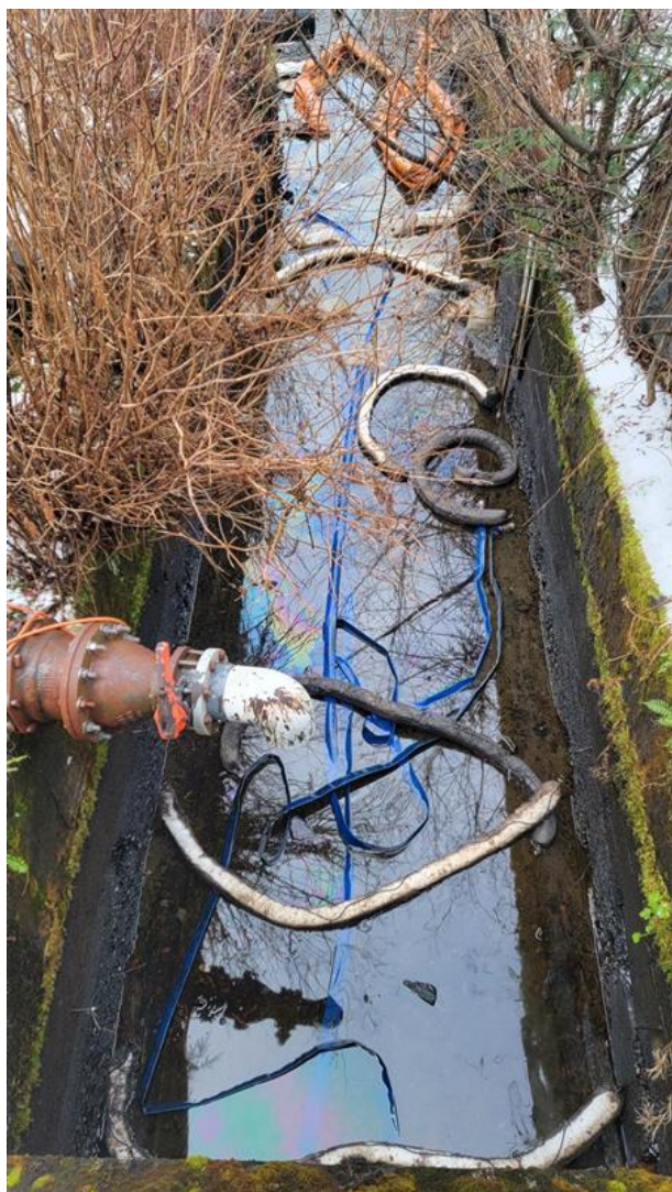
Photo taken by ADEC. November 18, 2021 Oil and sheen before it reaches the penstocks.
