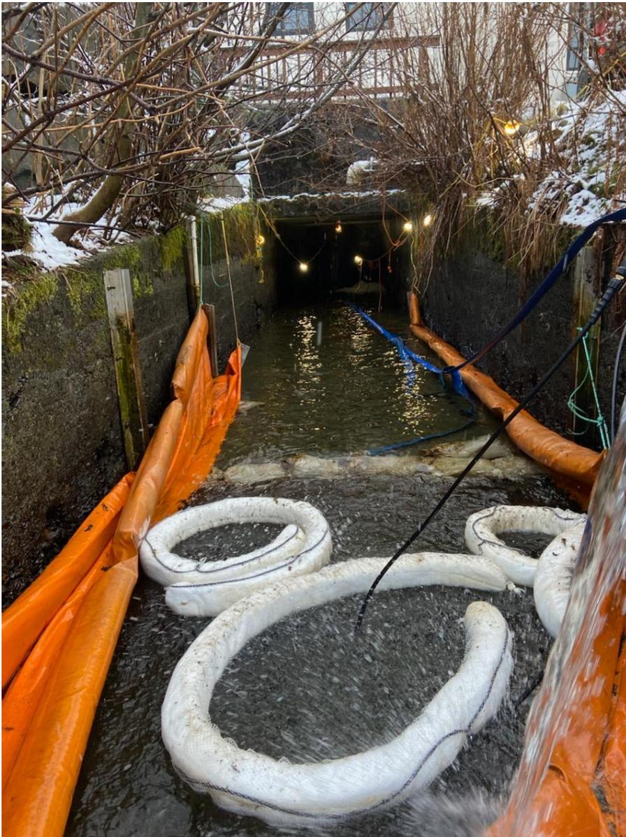
*Photo taken by MSD Sitka. November 23, 2021 Containment and sorbent boom deployed in outfall from the pond.*
