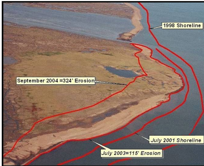
2 3 J.W. Dalton Drill Site Erosion. Located east of Utqiagvik on the Beaufort Sea near Teshekpuk Lake and Point Lonely DEW line site. 4 This photograph was taken in 2003; between the summers of 2003 and 2004 over 300 feet of shoreline eroded away along part 5 of the site. Approximately 600 feet of coastal plain were lost over a 6-year period. Photo provided by BLM
