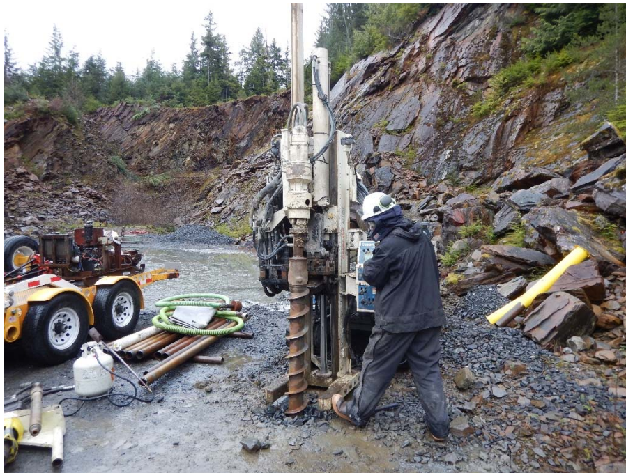
Photo 4: Advancement of borehole MW-02 with hollow-stem augers.
