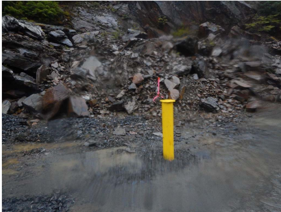
Photo 5: Installed security casing on MW-02. Date: 12/2/2016
