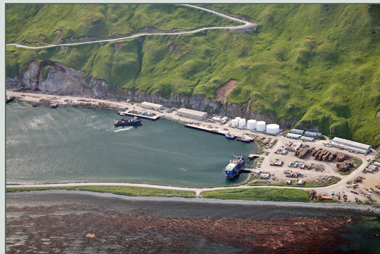
Dutch Harbor Processors looking northwest.
