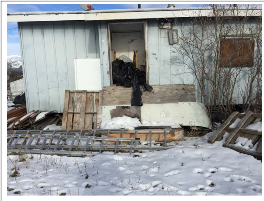
Photograph 1: Looking north at the former power plant. (September 22, 2015)
