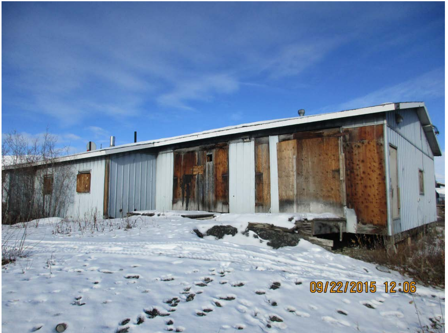
Figure 1 – The former Arctic Village Power Plant, in Arctic Village, Alaska.
