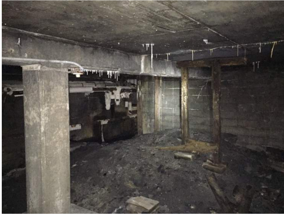
Figure A16 – Crawlspace floor beam with shoring.
