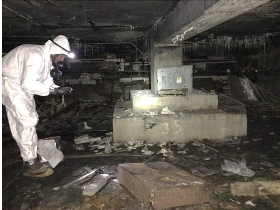
Figure A14 – Example of isolated column footing in crawlspace.
