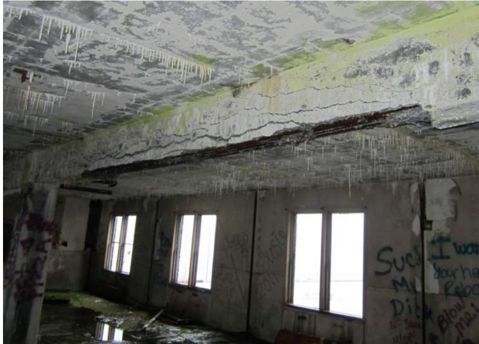
Figure A53 – Floor beam at 2 nd level Squad Room, northern half of Unit E. Beam is approaching collapse.
