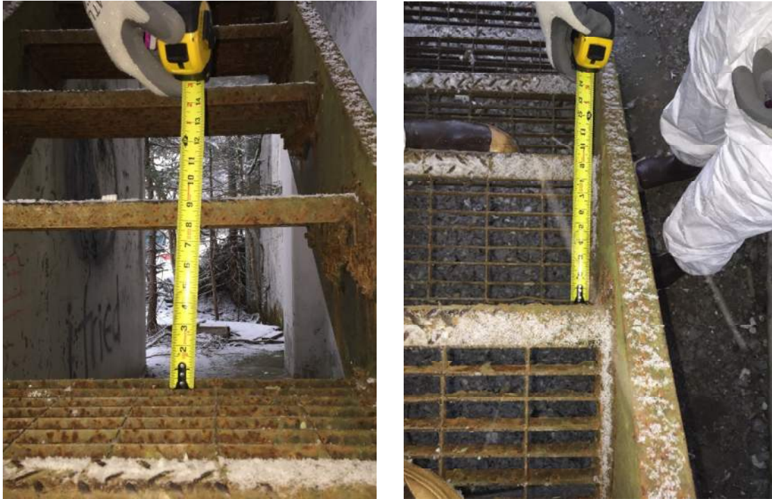
Figure A79 – Egress stair rise and run.
