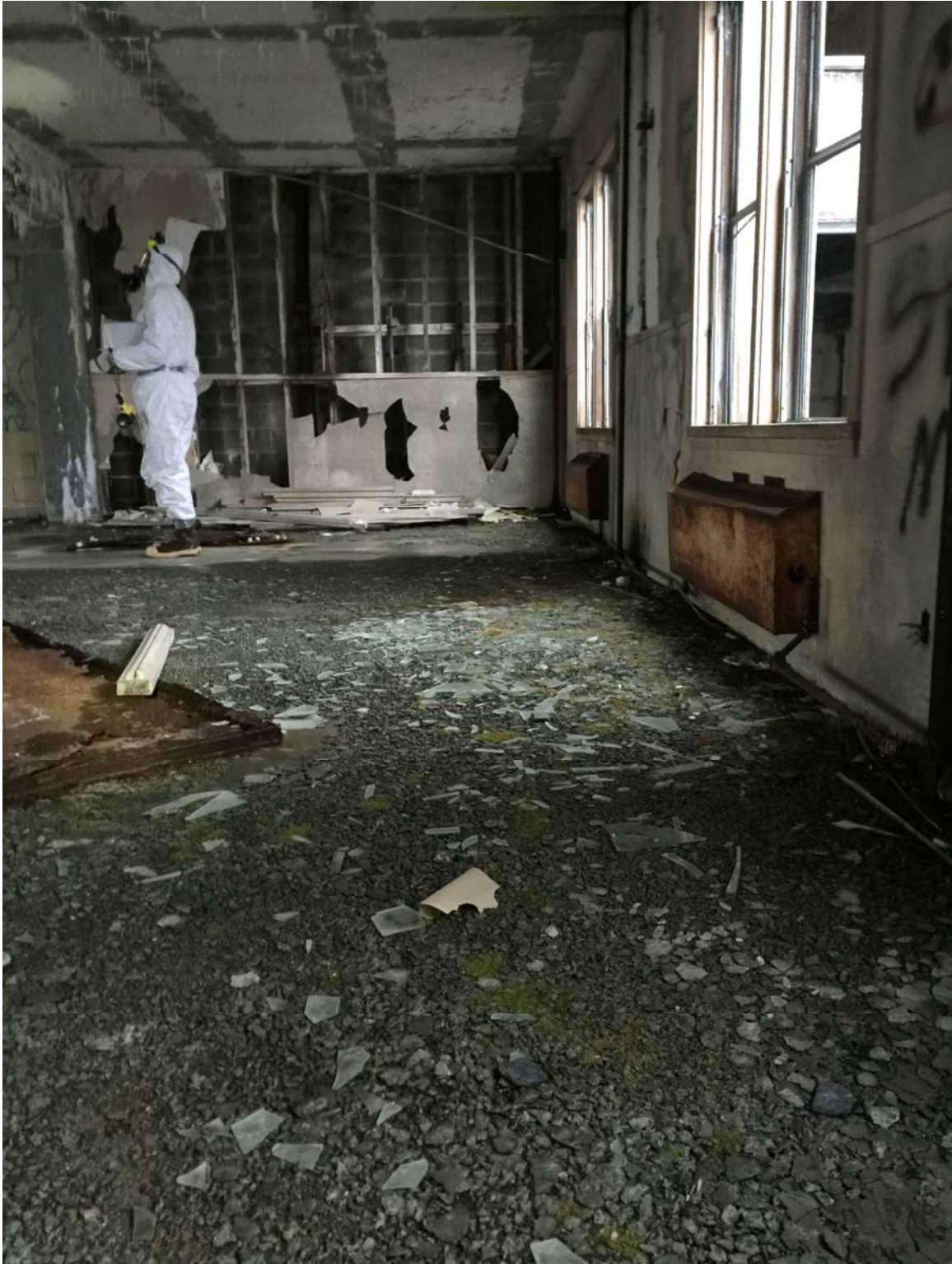
Figure A48 – Severely deteriorated 1 st floor slab adjacent to north facing windows.
