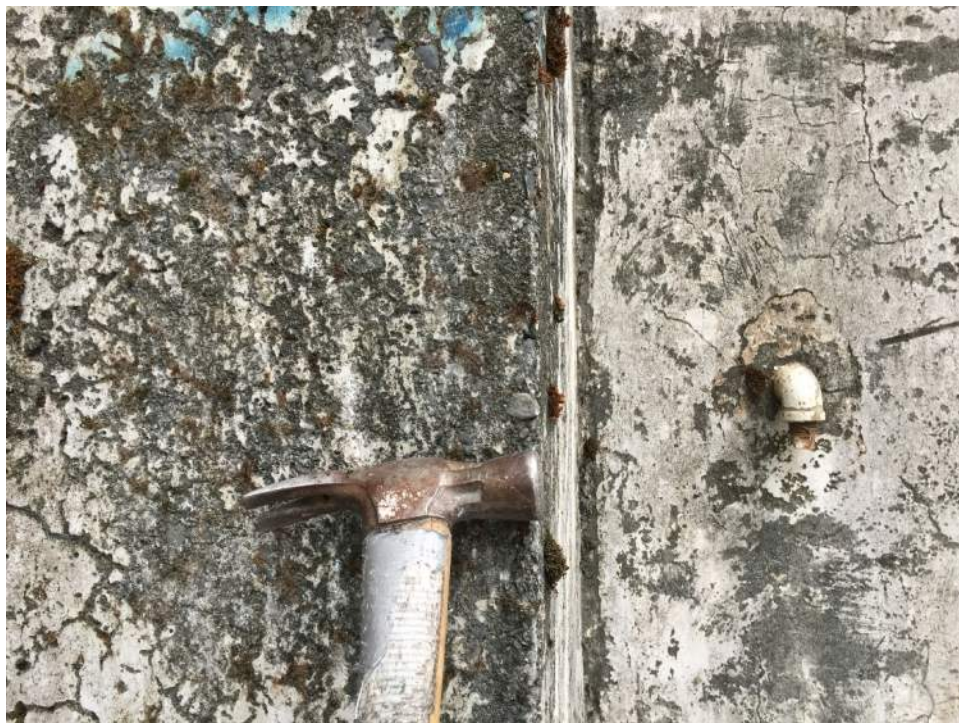
Figure A4 – Example of surface defect beneath moss growth on exterior wall
