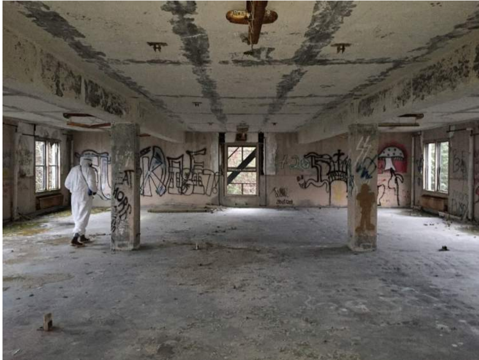
Figure A55 – Squad Room on southern end of Unit G’s 3 rd floor. This portion of the building is generally in the best condition.
