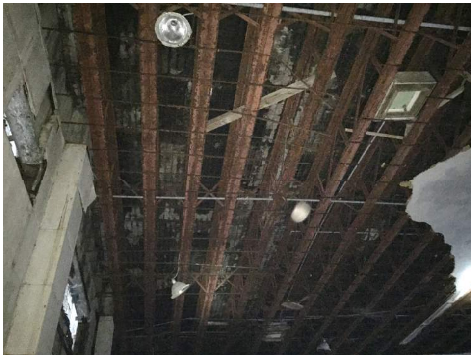
Figure A42 – Corroded steel open web roof joists at the theatre.
