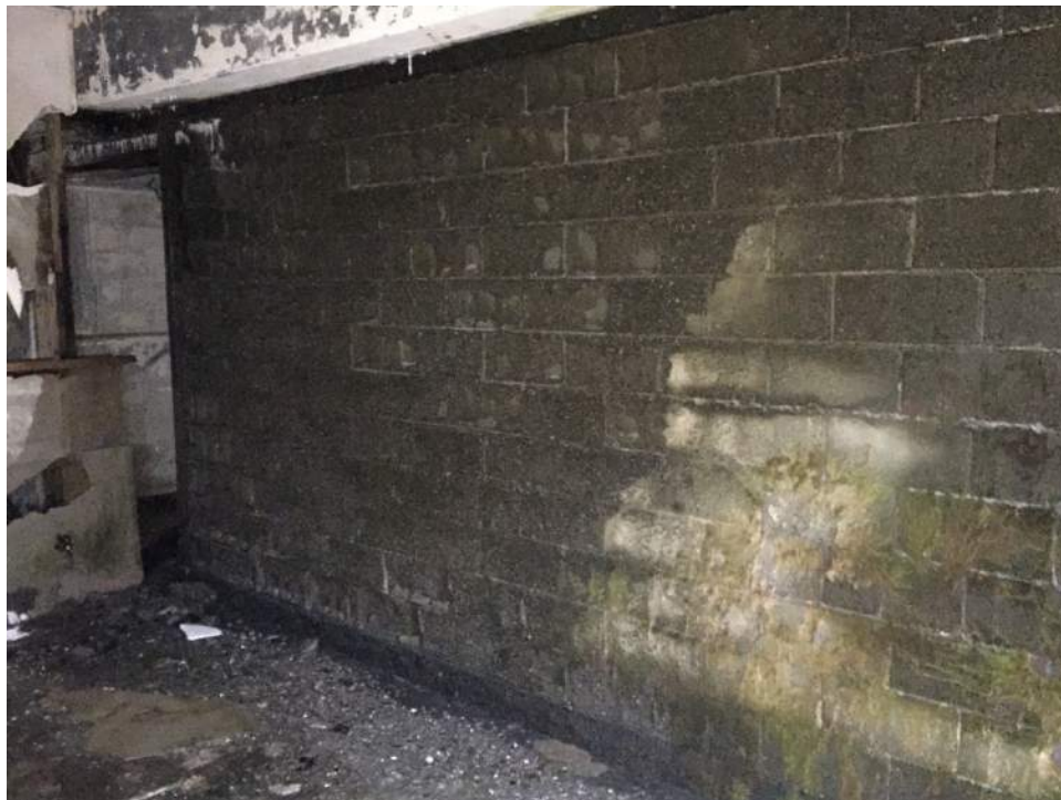
Figure A54 – Deteriorated CMU wall at the 2 nd floor level.
