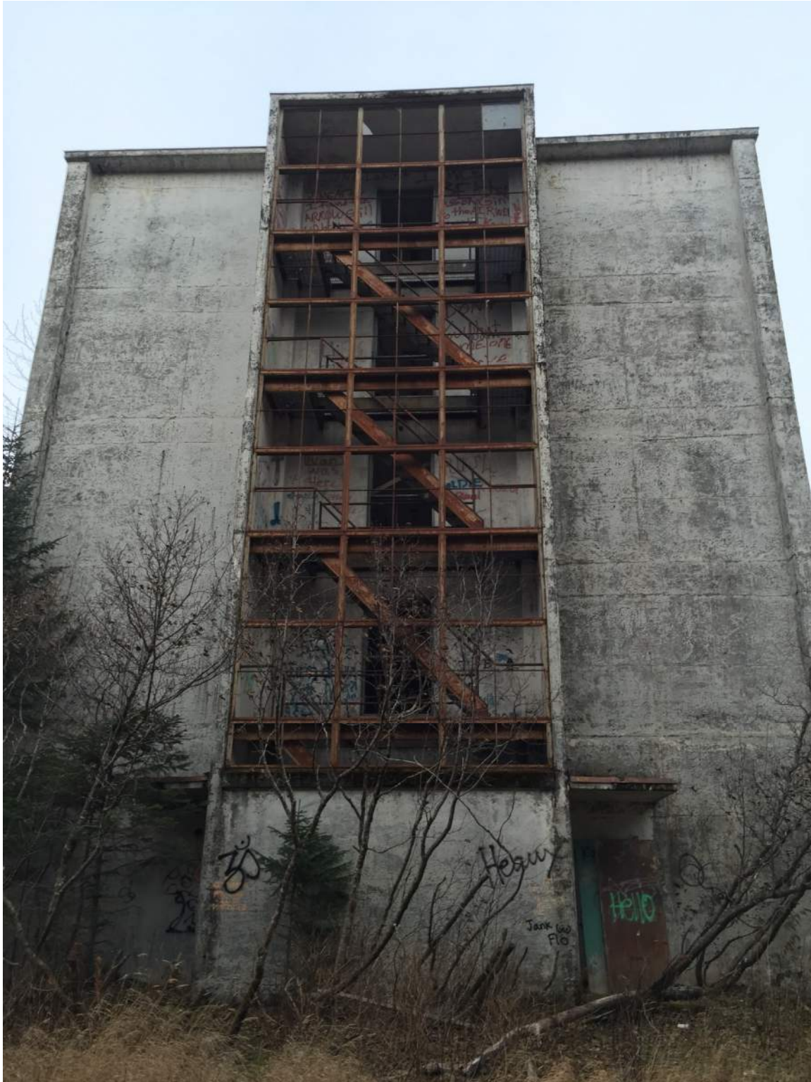
Figure A10 – Typical egress stair where curtain wall glass is gone and steel exposed to weather has corroded.
