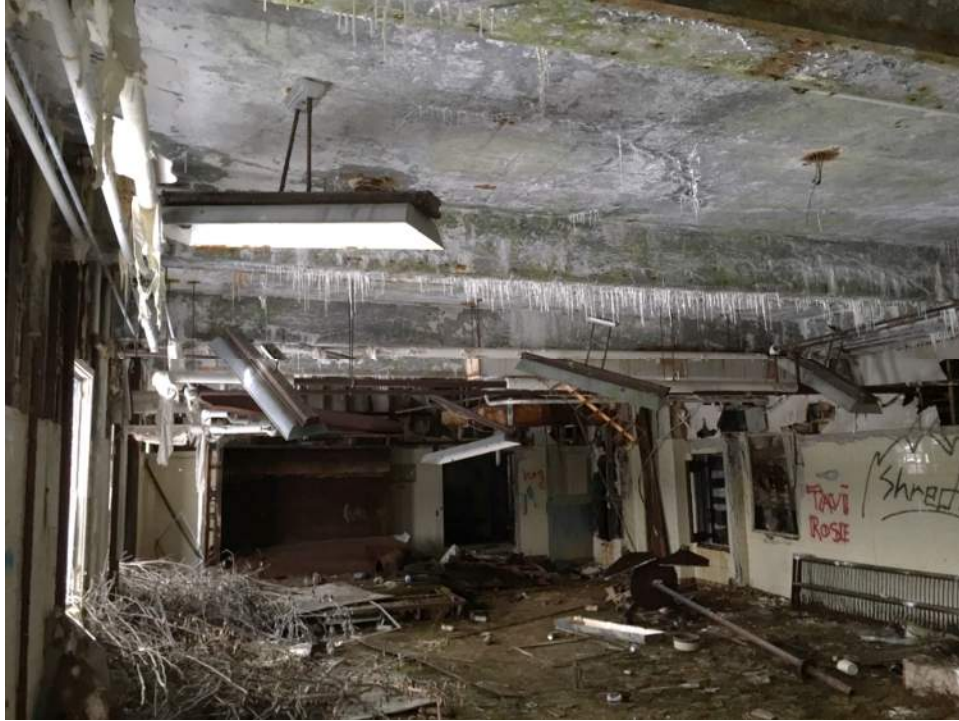
Figure A20 – Typical basement room with large amount of debris and stalactites hanging from floor beams and underside of floor slab above.
