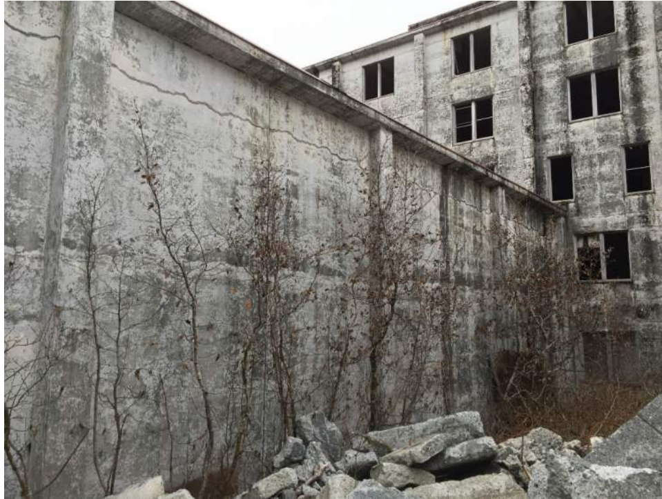
Figure A5 – East wall of theatre with large crack for the full wall length at approximate location of the roof joist bottom chord attachment.
