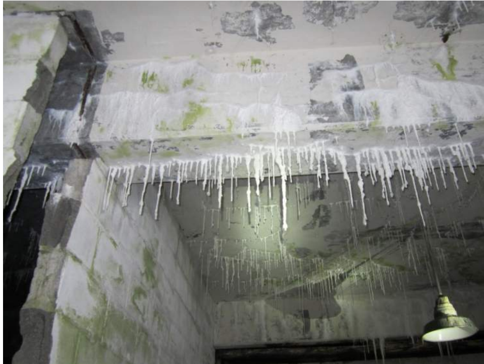
Figure A28 – Basement floor beam with stalactites and damaged CMU wall.
