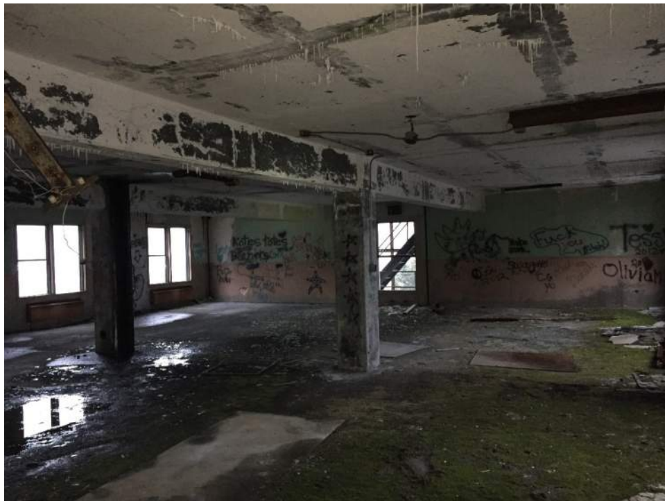
Figure A44 – Typical 1 st floor Squad Room.
