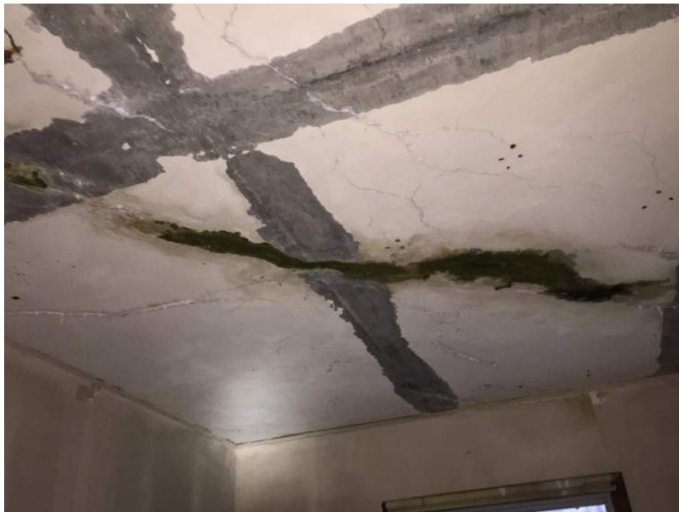
Figure A67 – Cracking in roof slab above 4 th floor barracks.
