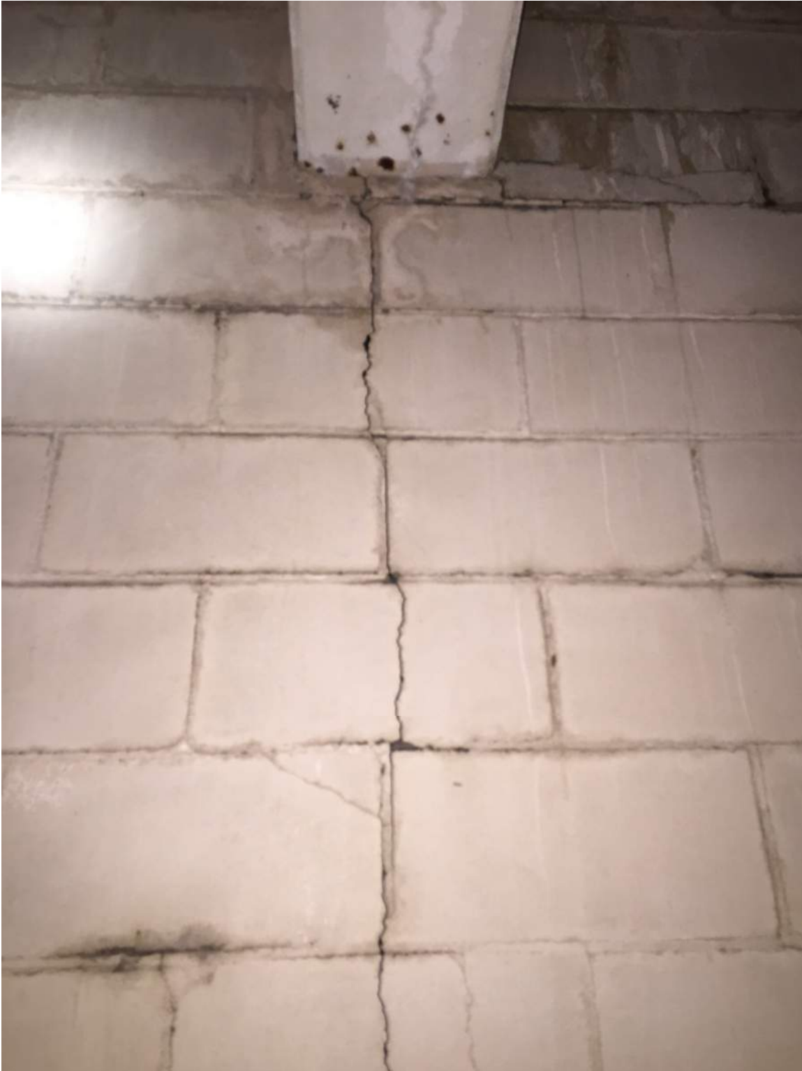
Figure A40 – Cracked CMU ground floor corridor wall at floor beam penetration.
