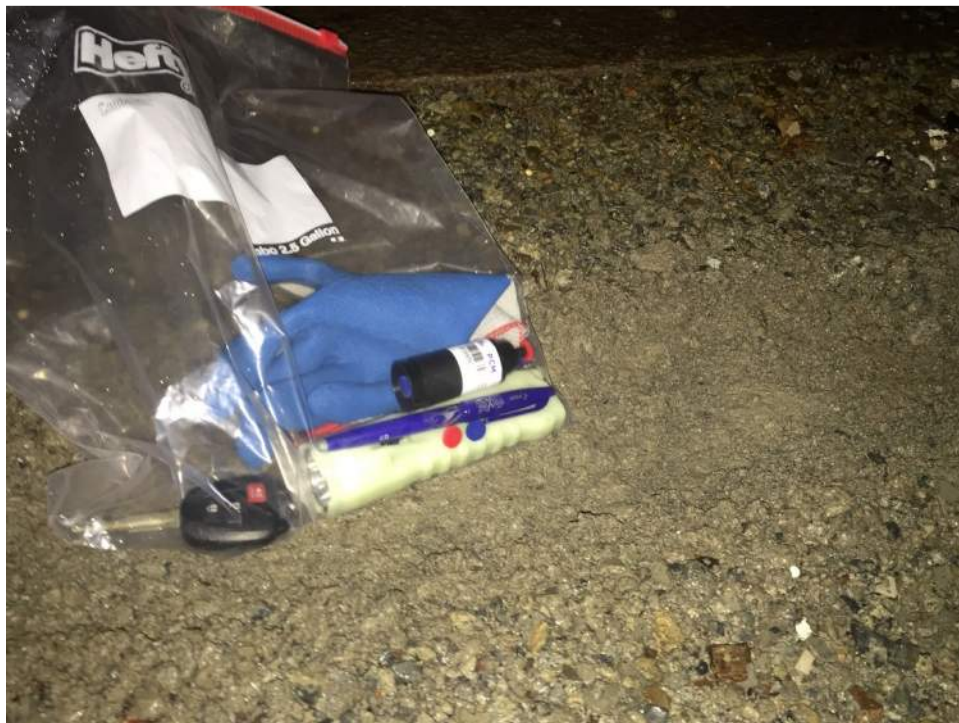
Figure A32 – Ground floor, close up of severely deteriorated slab surface.
