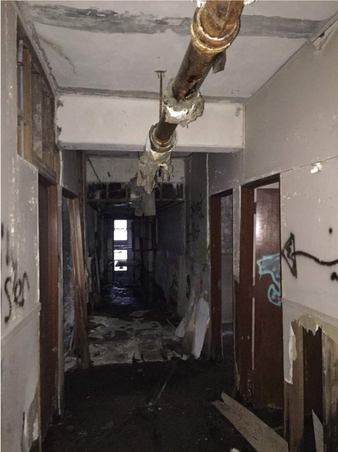
Figure A68 – 4 th floor corridor showing more architectural finishes still in place.
