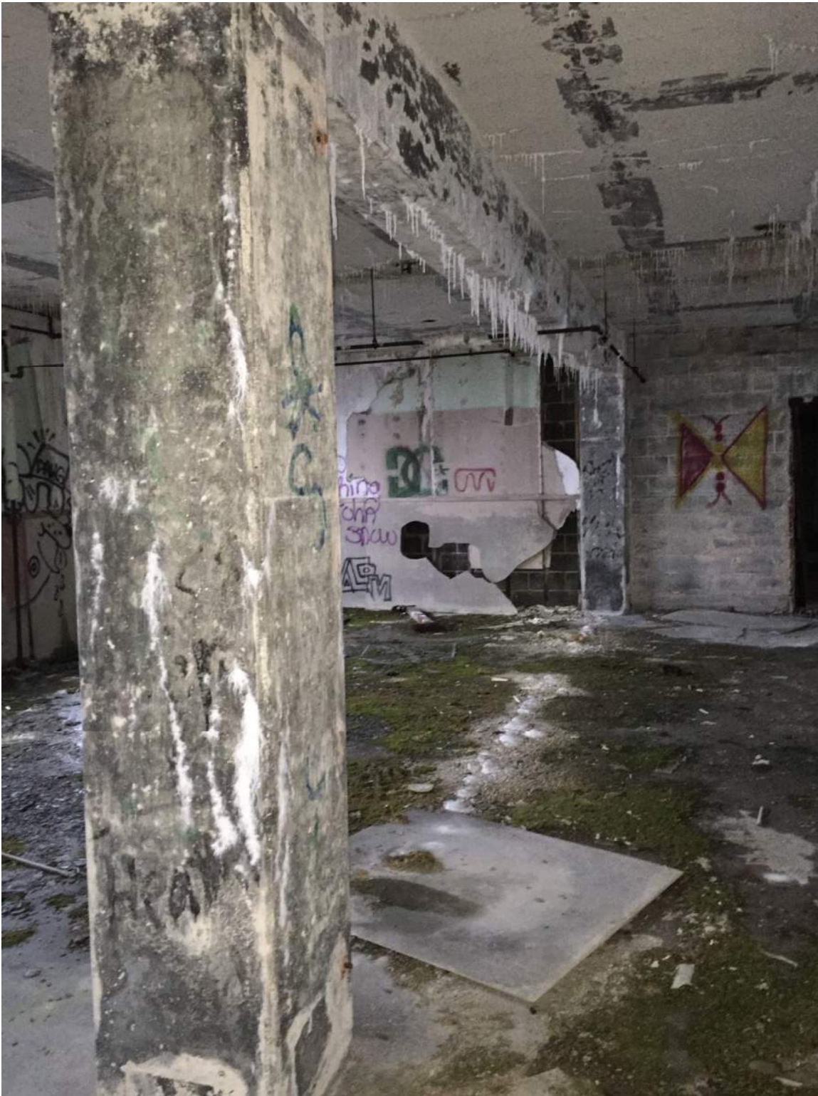
Figure A57 – 3 rd floor Squad Room on northern half of unit. Stalactites and stalagmites are present along beam line.
