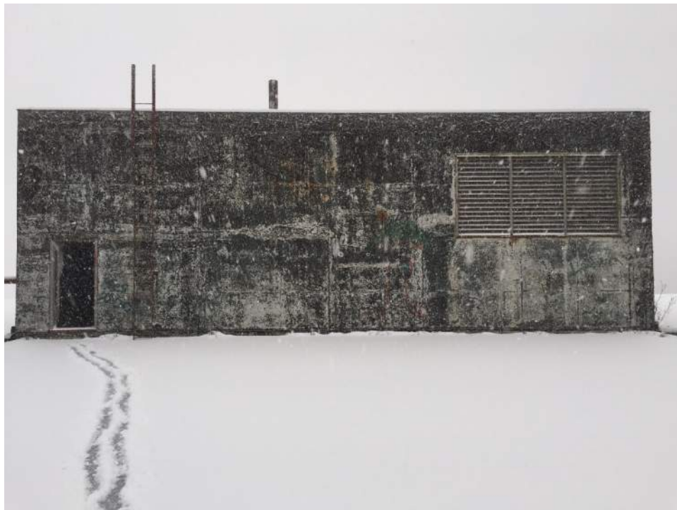
Figure A74 – Typical penthouse fan room.
