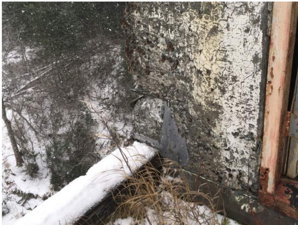
Figure A76 – Shallow surface defects of concrete penthouses, typical.
