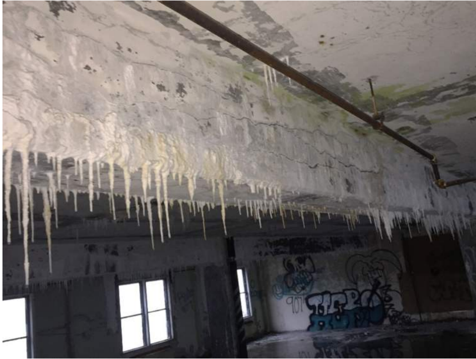
Figure A60 – 3 rd floor beam with horizontal cracking along beam face.
