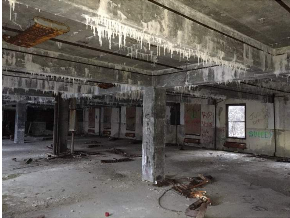
Figure A43 – Typical 1 st floor Day Room.
