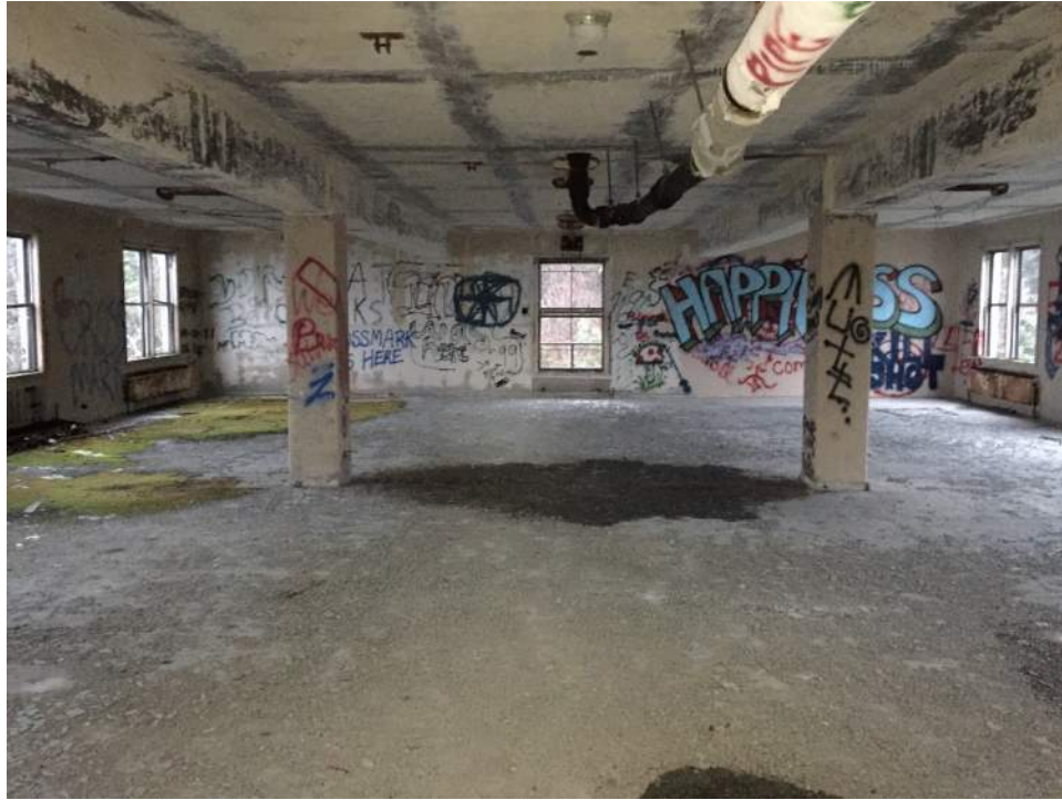
Figure A63 – Squad Room on southern end of Unit G’s 4 th floor. This portion of the building is generally in the best condition.
