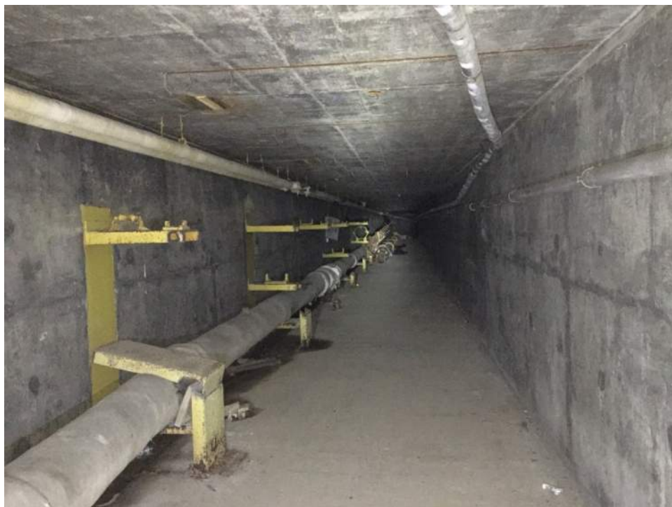
Figure A19 – Utilidor tunnel.
