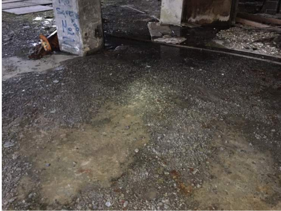
Figure A31 – Ground floor, elevated slab with severe spalling.
