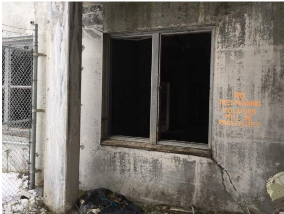
Figure A6 – Concrete shear wall with diagonal crack protruding from upper left and lower right window corners.
