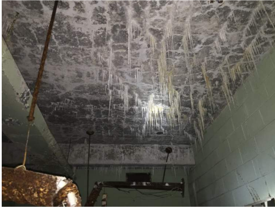
Figure A24 – Basement ceiling with large stalactite concentrations.
