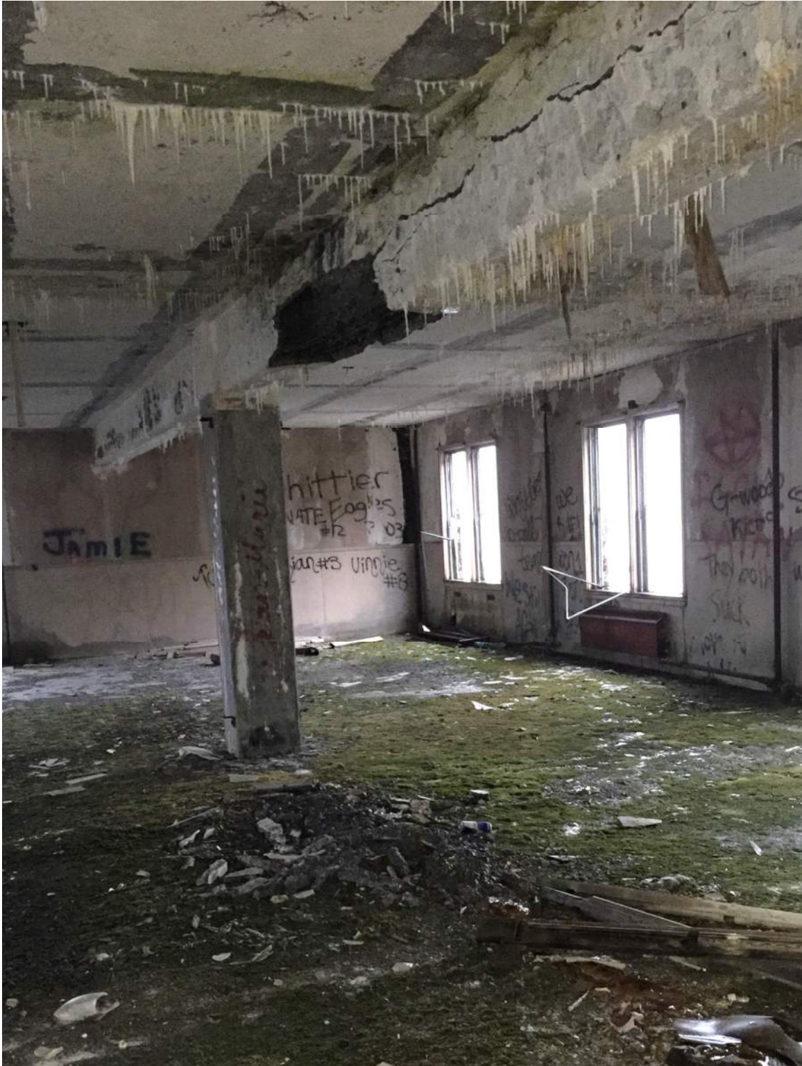
Figure A52 – Floor beam at 2 nd level Squad Room, northern half of Unit G. Beam is approaching collapse.
