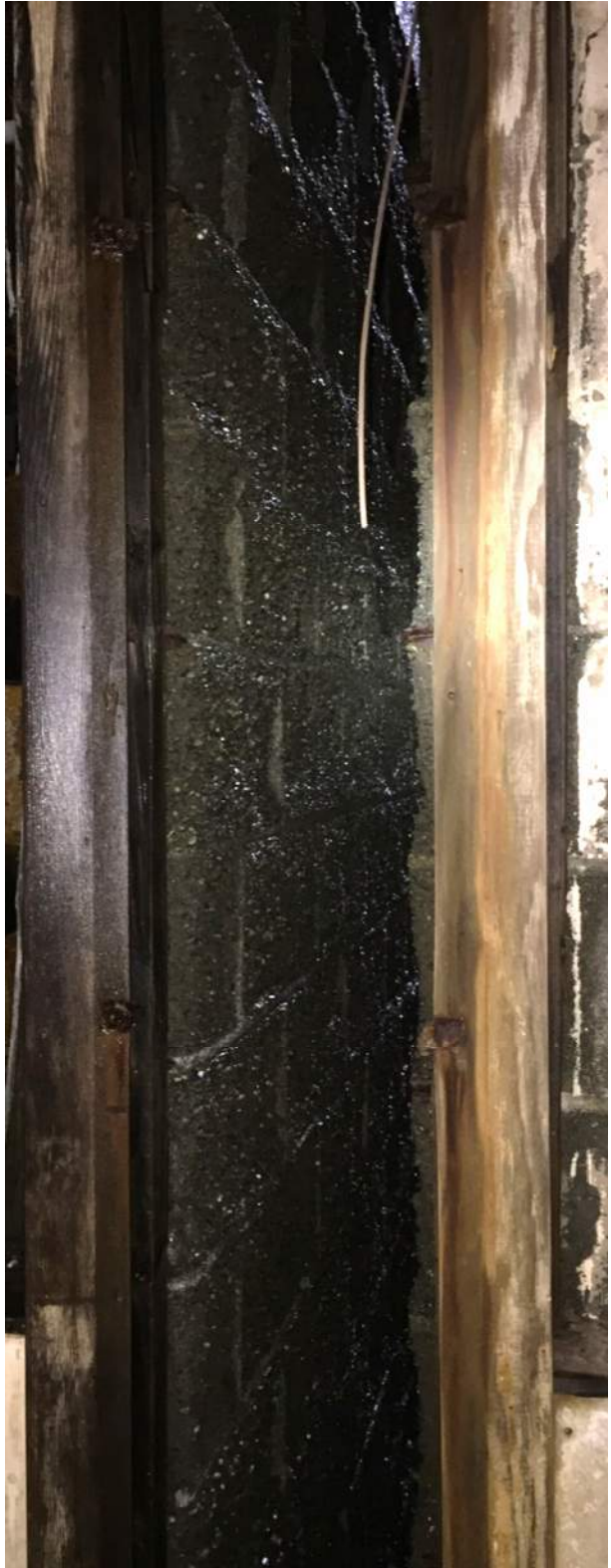
Figure A39 – Ground floor CMU, extremely deteriorated at seismic joint.
