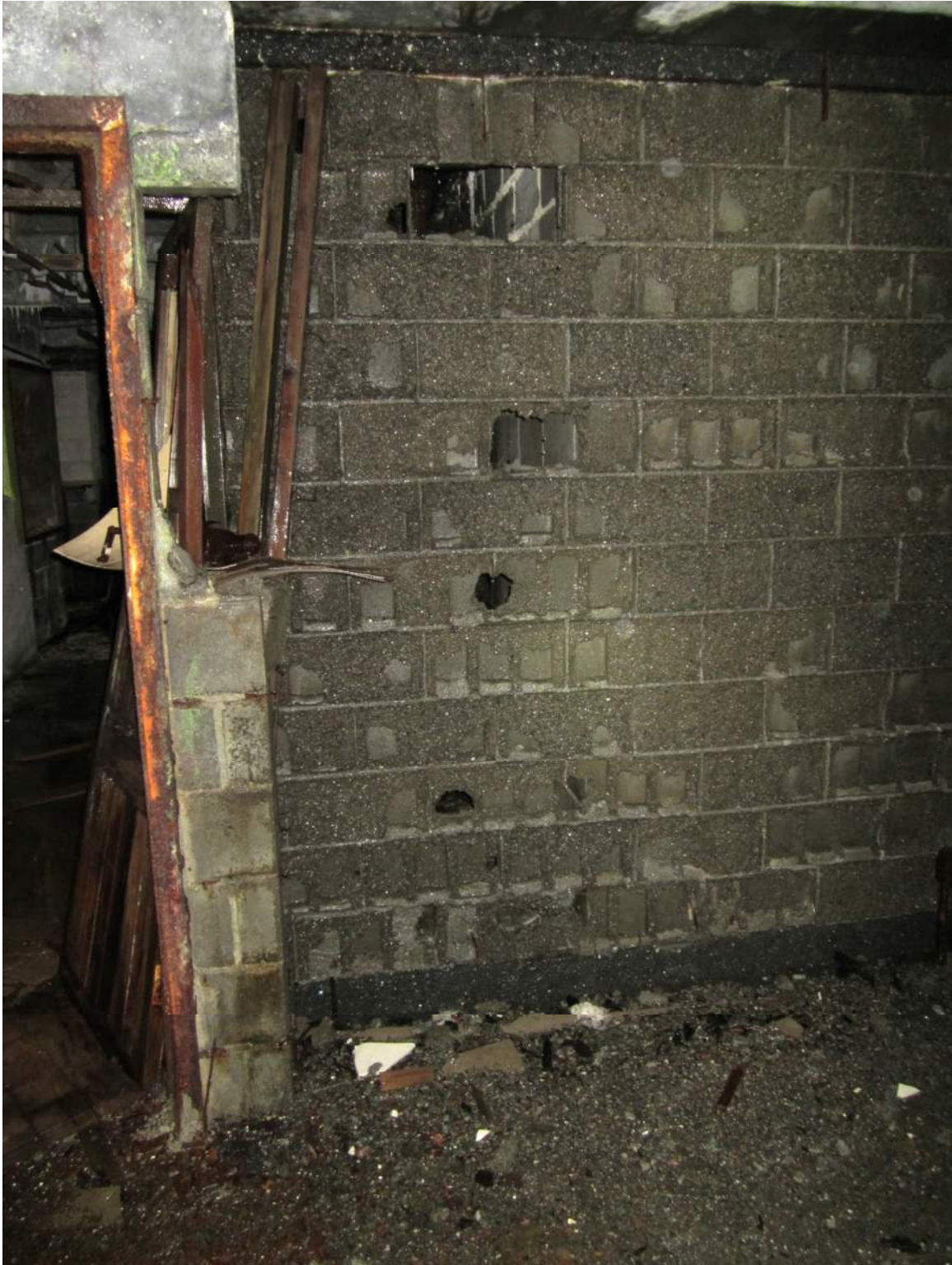
Figure A62 – Severely deteriorated CMU wall at 3 rd floor level.
