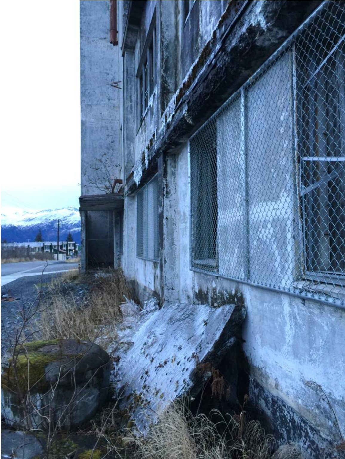
Figure A11 – Collapsed portion of concrete canopy on north façade.
