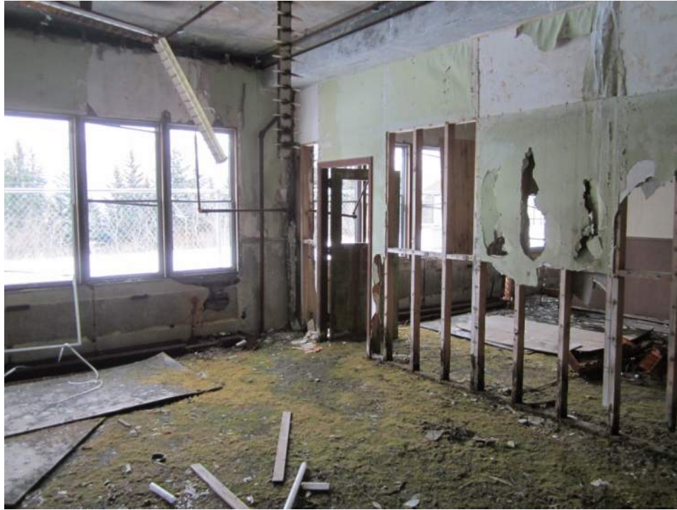
Figure A26 – Daylight basement with debris and significant moss growth on floor.
