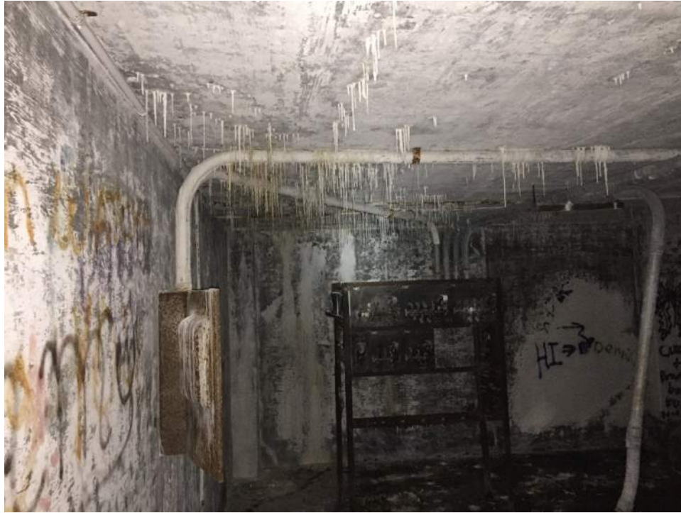
Figure A77 – Typical penthouse mechanical mezzanine. Stalactites visible from the ceiling slab.
