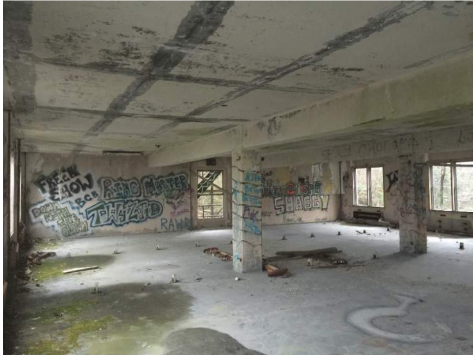
Figure A51 – Squad Room on southern end of Unit G’s 2 nd floor. This portion of the building is generally in the best condition.
