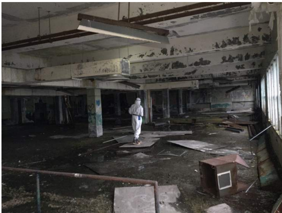
Figure A29 – Mess hall at the north side of the ground floor.
