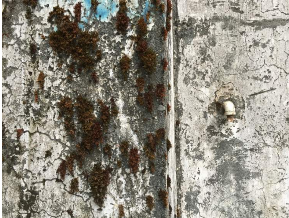
Figure A3 – Example of moss growth on exterior wall.
