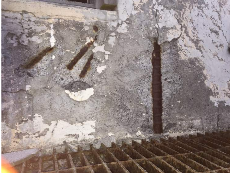
Figure A7 – Example of exposed exterior wall rebar at egress stair landing.
