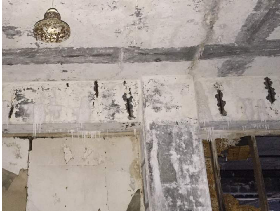
Figure A36 – Ground floor beam/column connection with exposed beam stirrups and stalactites.
