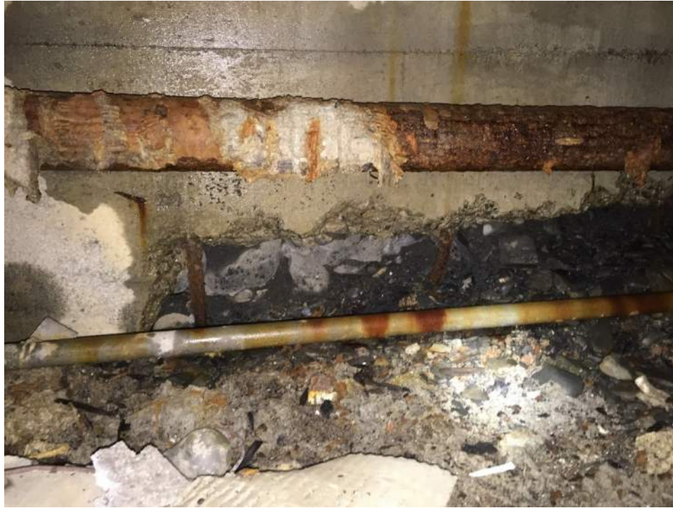
Figure A18 – Wall in crawlspace with vertical rebar doweled directly to rock.
