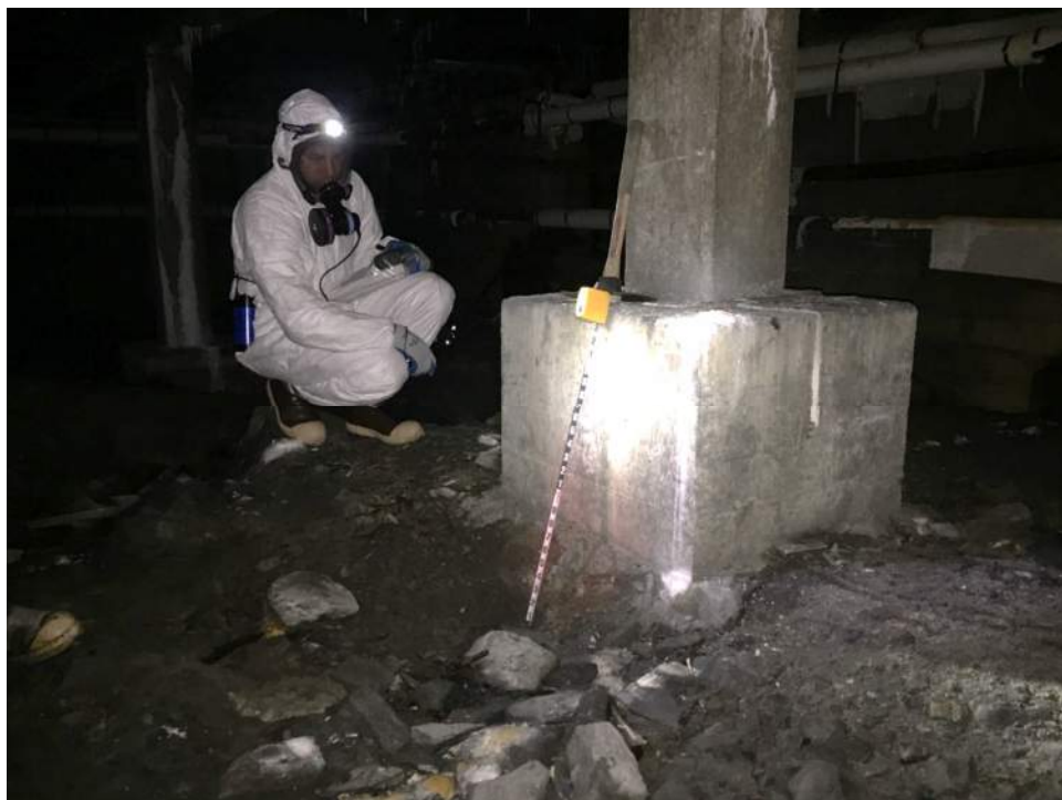
Figure A15 – Column pedestal cast directly on rock in crawlspace.
