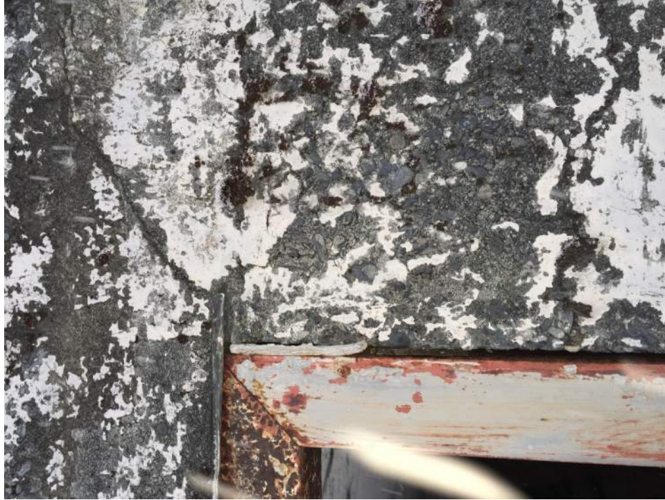
Figure A75 – Shallow surface defects of concrete penthouses, typical.
