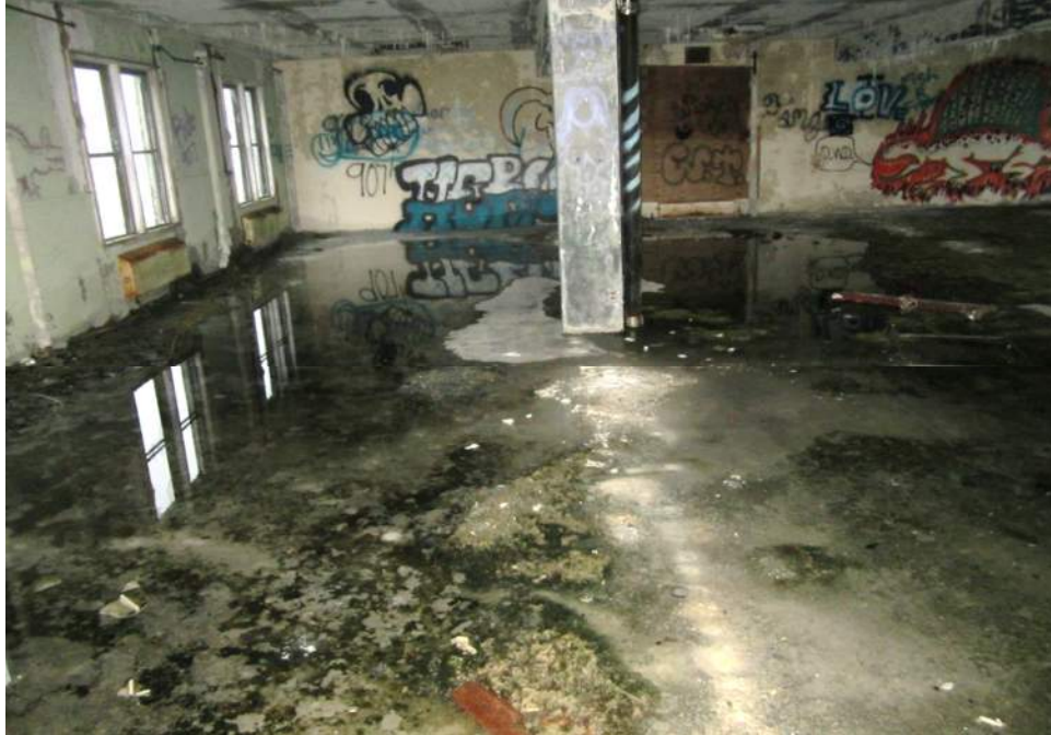
Figure A58 – Flooded 3 rd floor Squad Room. Stalagmites forming on floor along the beam line.
