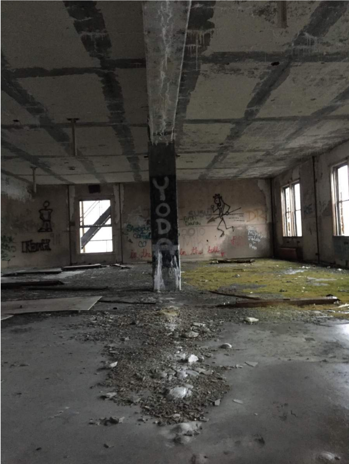
Figure A47 – Beam/column grid at 1 st floor Day Room with stalactites suspended from beam and stalagmites beginning to form on the floor slab.
