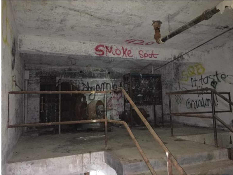
Figure A73 – Interior of Unit A fan room, accessed via stair 2.
