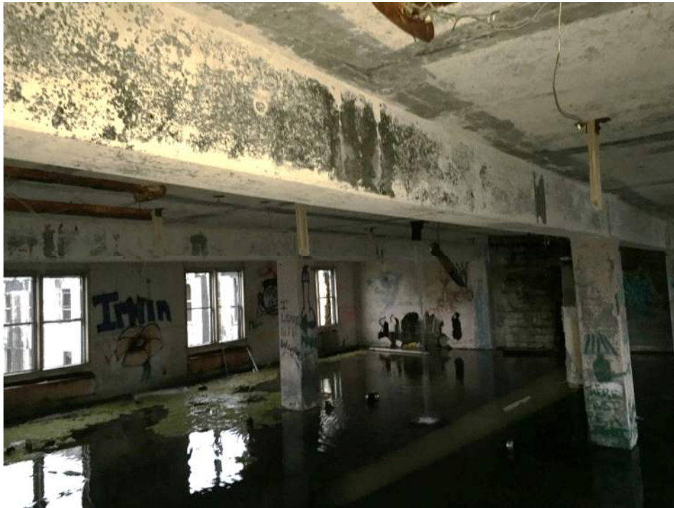
Figure A64 – Flooded squad room on norther side of the building.
