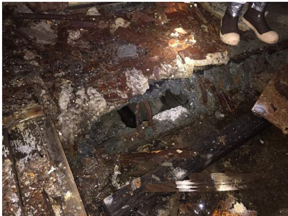
Figure A23 – Hole in bowling alley floor to crawlspace below.
