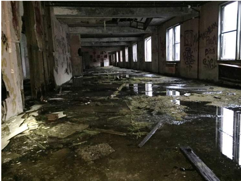
Figure A59 – 3 rd floor lounge/game room with flooded floor.
