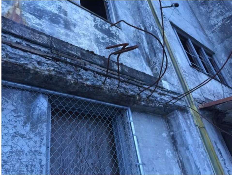
Figure A12 – Edge beam with rebar protruding from collapsed canopy.
