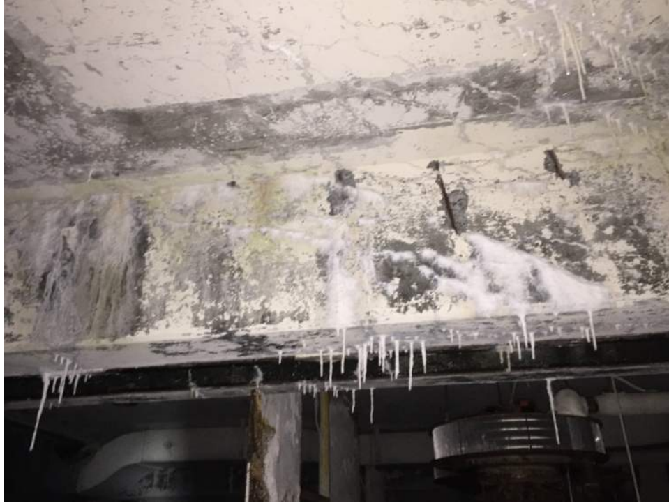
Figure A66 – Close up of deteriorating roof beam with exposed stirrups.
