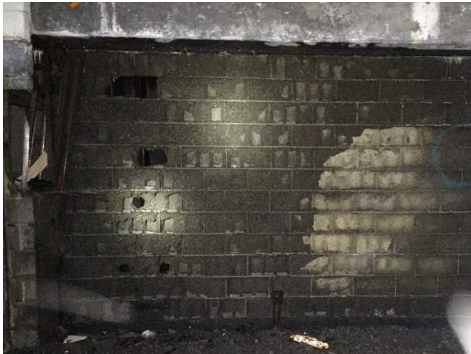
Figure A50 – Severely deteriorated CMU at 1 st floor, with holes eroded complete through.
