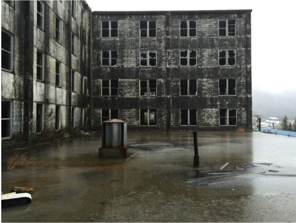
Figure A69 – Low roof over Mess Hall and Kitchen.
