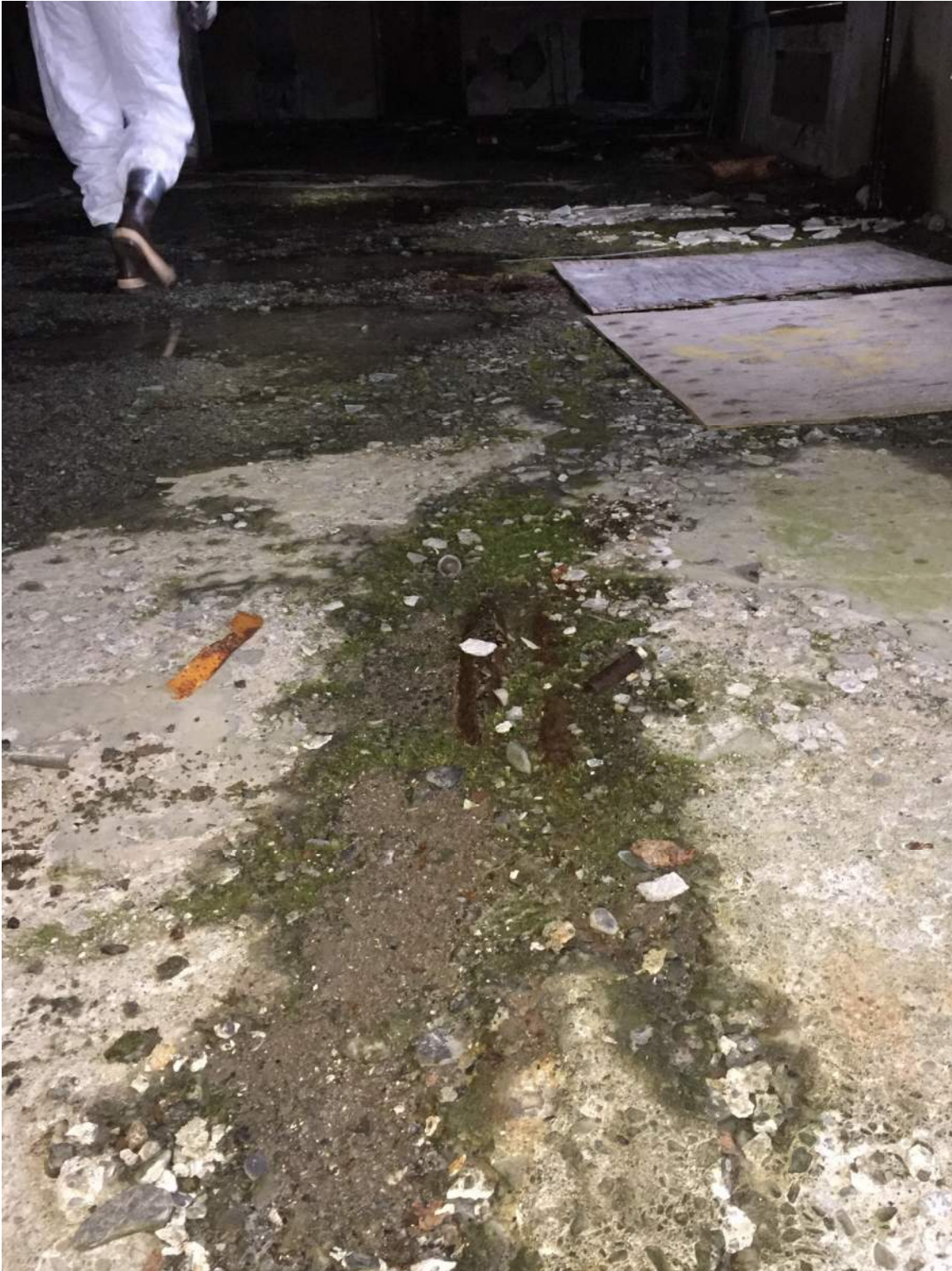
Figure A33 – Pipes embedded ground floor slab that have ruptured from frozen water and damaged the floor slab.
