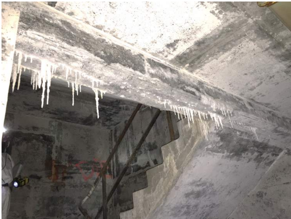
Figure A78 – Stairwells to for roof access were typically in fair condition, but not free of defects.
