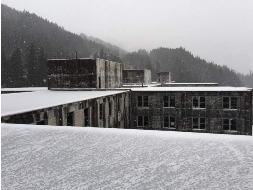
Figure A71 – Penthouse fan rooms for Units A, C and E.
