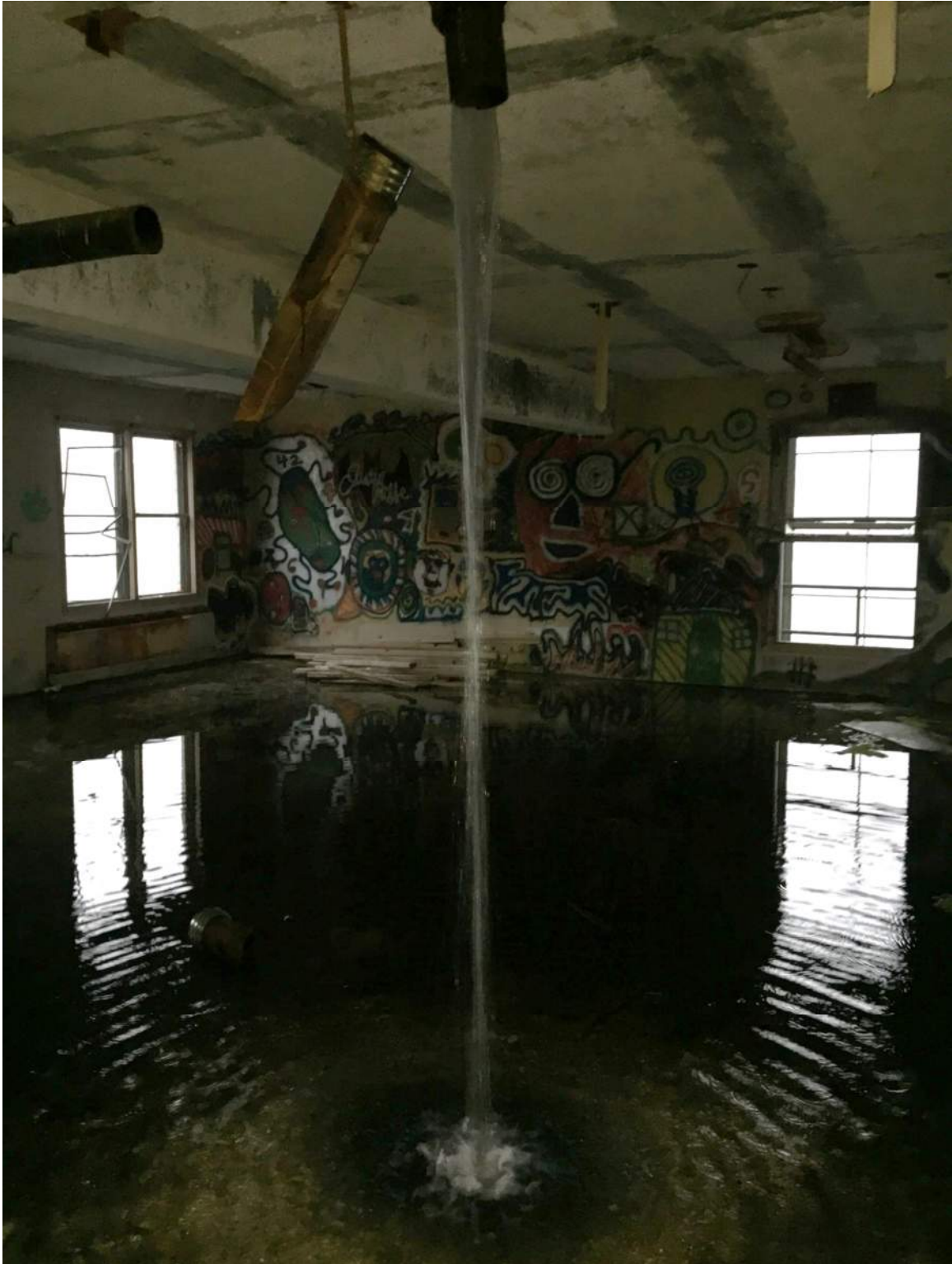
Figure A65 – Broken rain leader draining directly onto floor slab.
