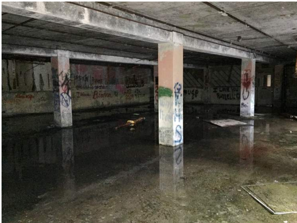
Figure A46 – Flooded 1 st floor room.
