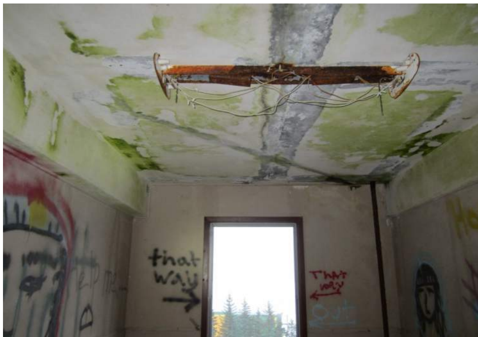
Figure A61 – 3 rd floor barracks with architectural finishes still intact (although damaged).
