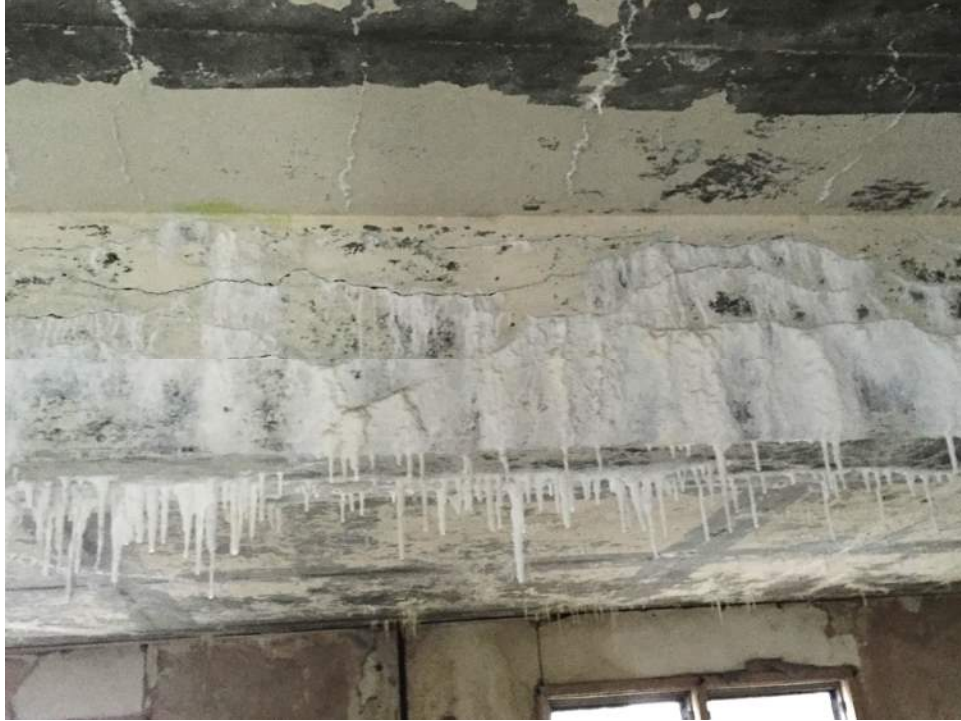
Figure A49 – Close up of stalactites and calcium carbonite forming on the side of the concrete beam, through large horizontal cracks.
