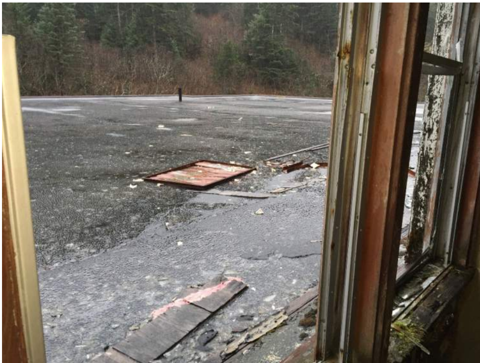
Figure A70 – Low roof over the theatre.
