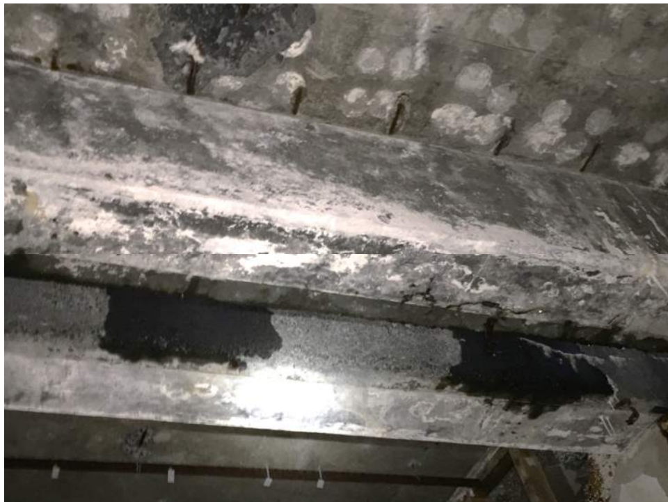
Figure A35 – Ground floor, exposed slab reinforcement.
