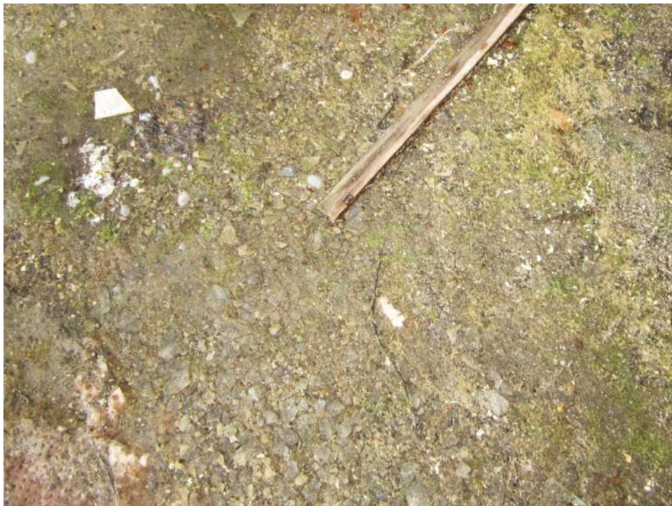
Figure A27– Close up view of basement floor with moss growth and spalled concrete slab surface.
