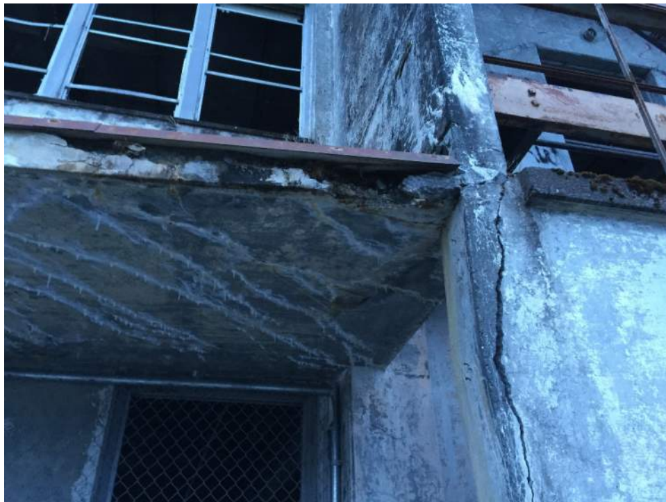
Figure A13 – Large crack at concrete wall / canopy attachment. Failure appears imminent.
