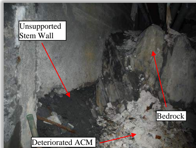
Stem wall observed in a utility tunnel near northwest corner of Unit G.
