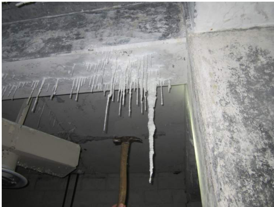
Figure A25 – Long stalactite on underside of floor beam.
