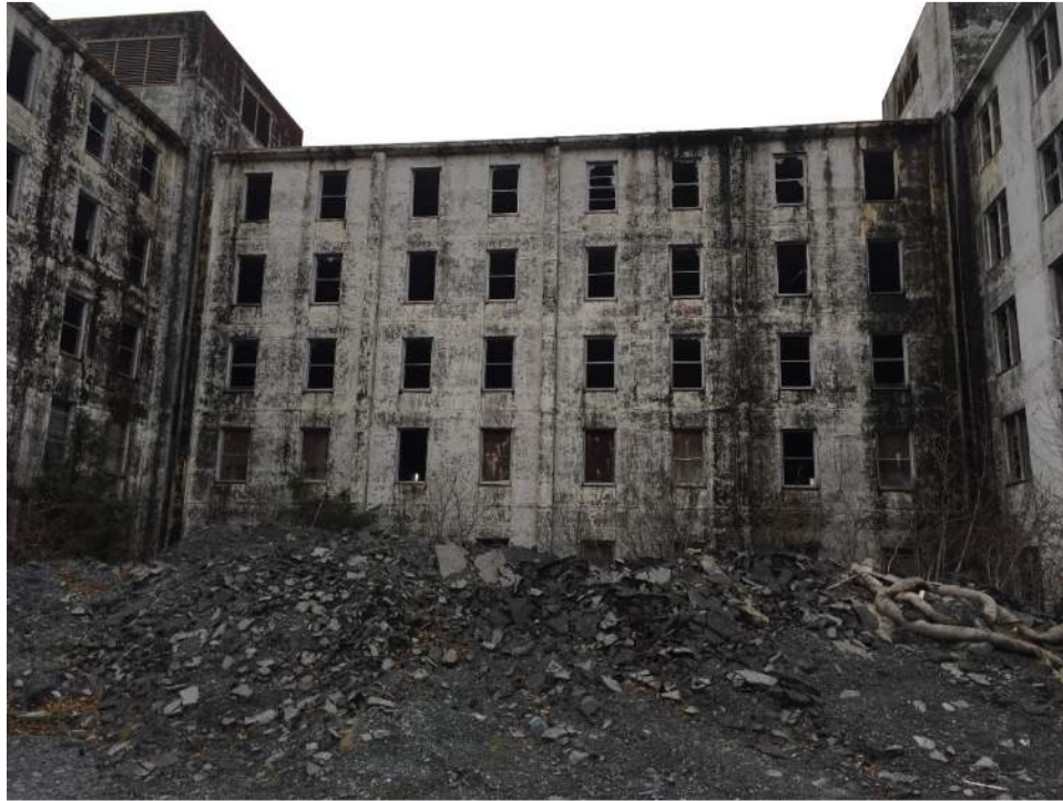
Figure A1 – Typical southern building elevation with perforated concrete shear walls and missing windows
