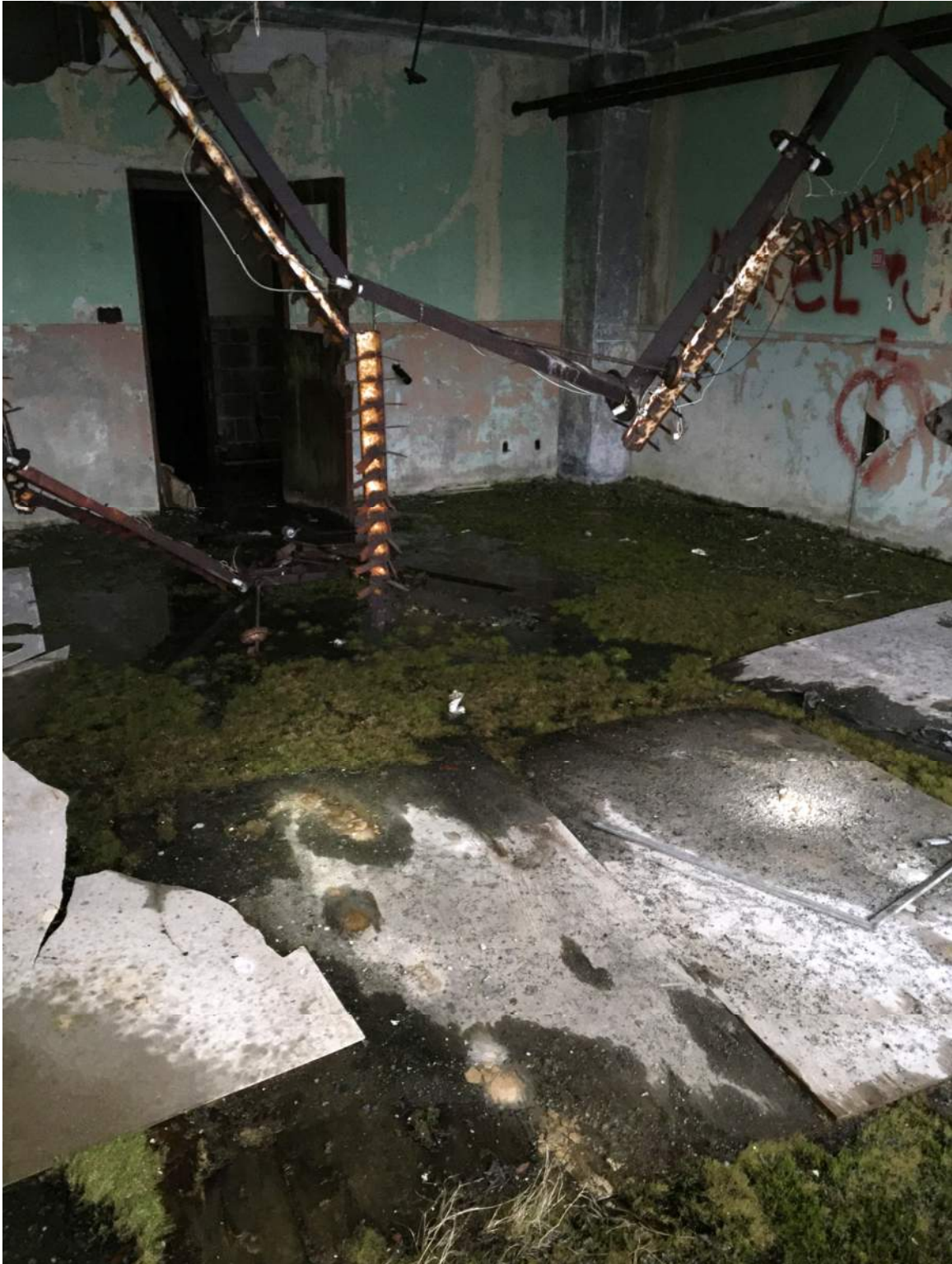
Figure A30 – Typical ground floor office with floor flooded from water infiltration and heavy moss growth on slab.
