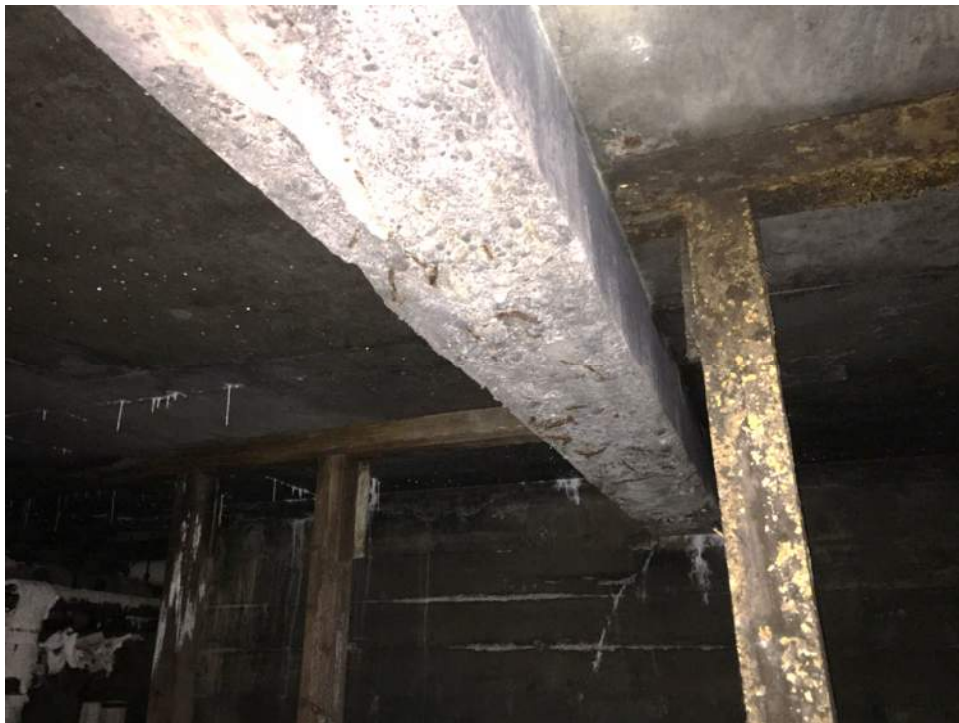
Figure A17 – Crawlspace floor beam with voids on underside and exposed rebar.
