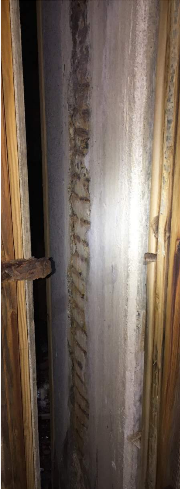
Figure A38 – Ground floor column at seismic joint with exposed spiral ties.
