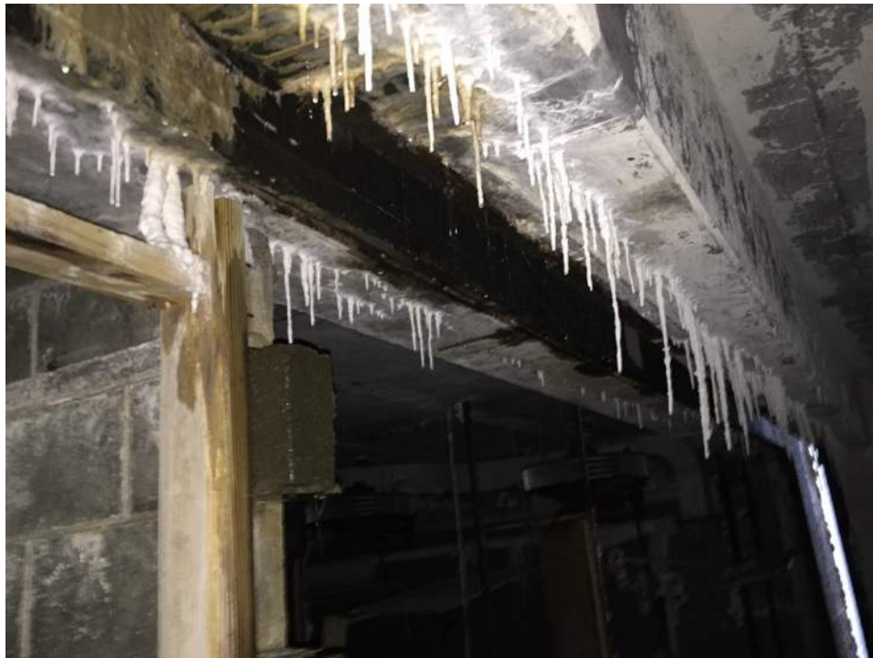
Figure A56 – Seismic joint with 3 rd floor beams each side. Stalactites present on each beam and flashing is missing at joint.
