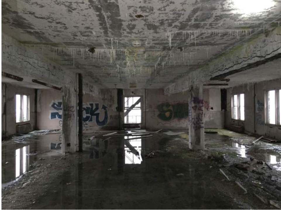
Figure A45 – 1 st floor day room with beam each beam line extremely deteriorated.
