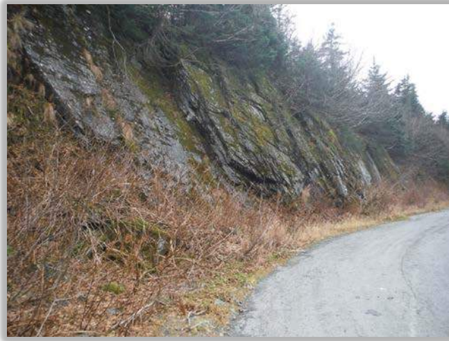
Excavated rock slope behind the northeast corner of the building. Looking southwest.
