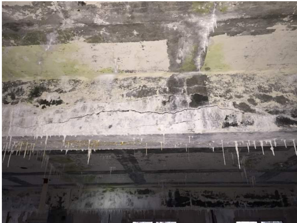
Figure A51 – 2 nd floor beam with large horizontal cracks.
