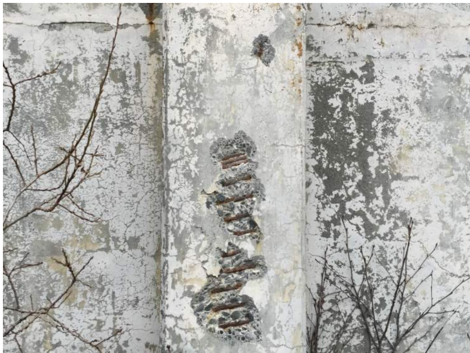
Figure A8 – Example of exterior concrete column with exposed, corroded spiral ties.
