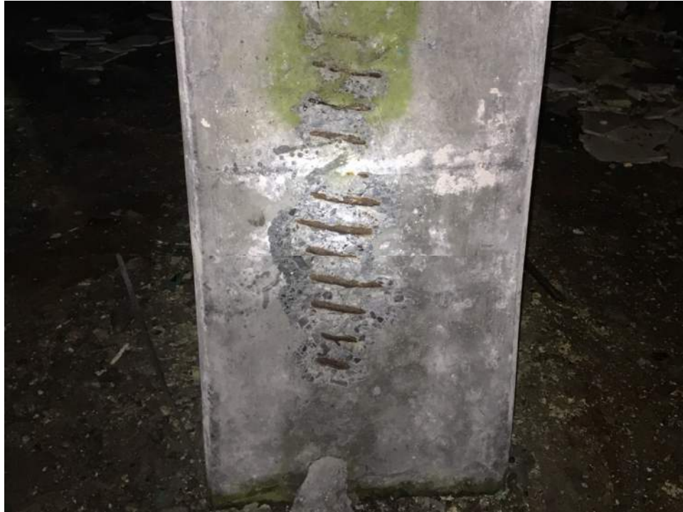
Figure A34 – Ground floor interior column with exposed ties.
