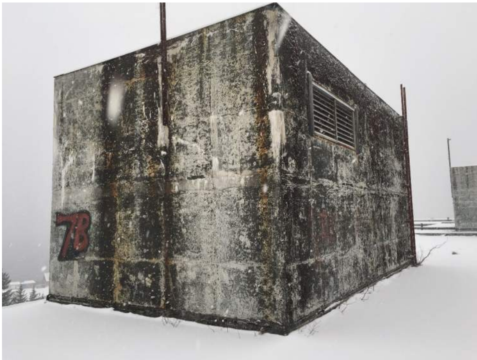
Figure A72 – Smaller penthouse fan room at Unit A.
