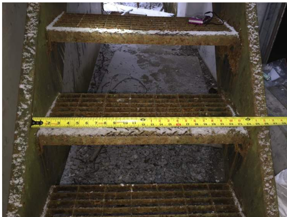
Figure A80 – Egress stair width.
