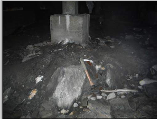
Typical footing observed in the sub-basement area of Unit A. Note potential in-situ bedrock exposed in foreground.
