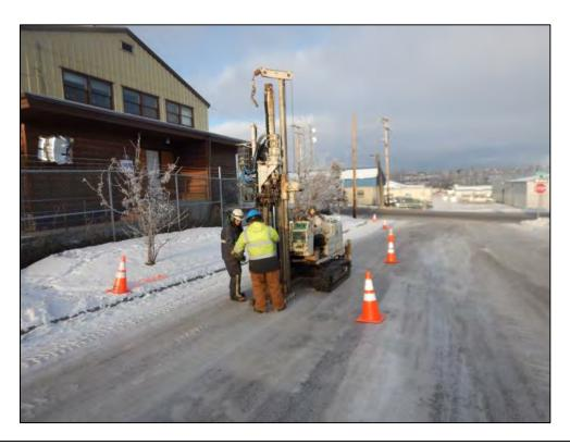
Photograph 1: Looking north. Geotek personnel performing vapor monitoring well installation.
