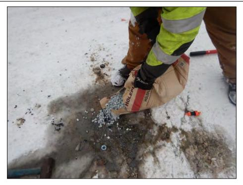
Photograph 5: Filling empty borehole with bentonite chips.
