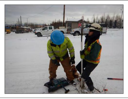
Photograph 4: Looking east. Removal of a vapor monitoring well.
