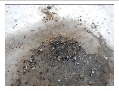
Photograph 6: Close up of asphalt patch applied during decommissioning.
