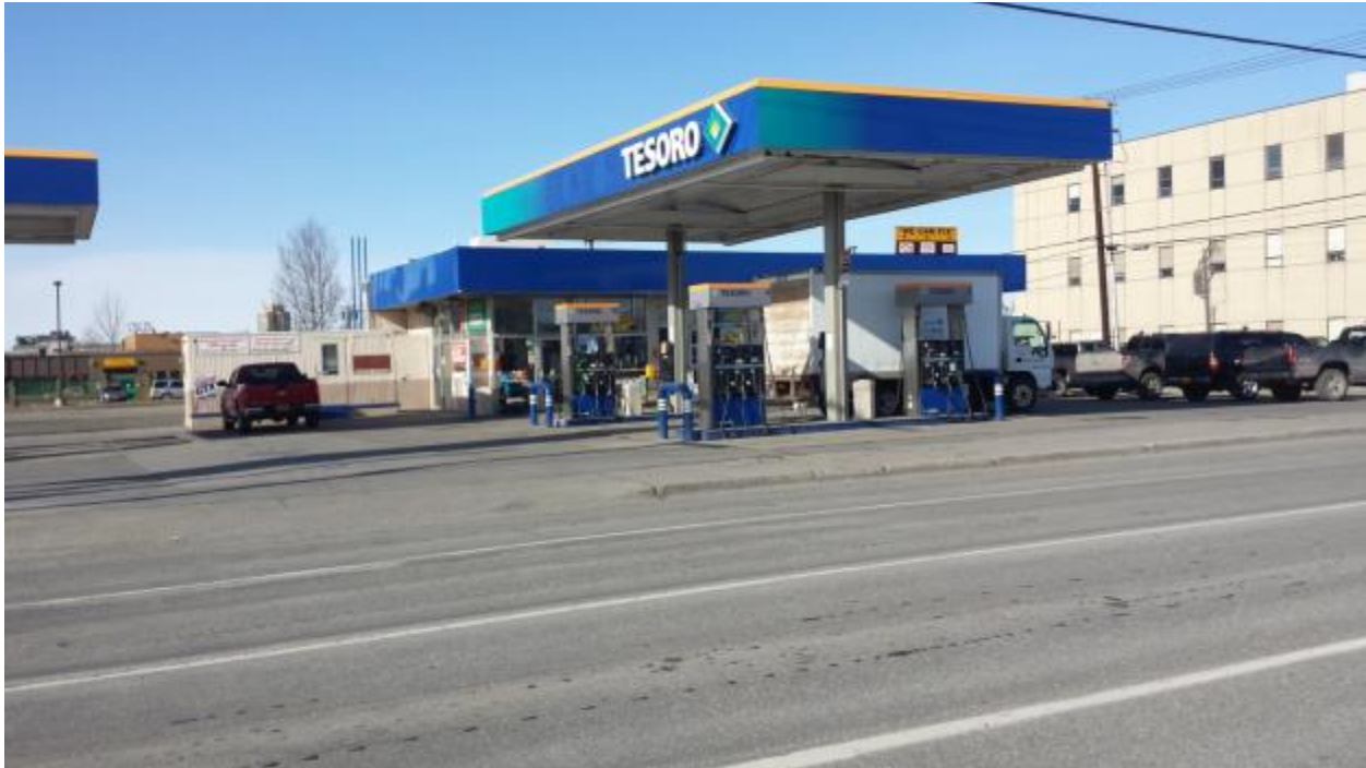
13. Tesoro gas station, known historic contamination at this property
