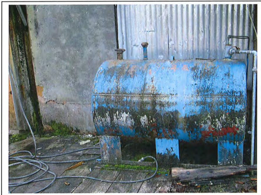
Photo 8: Active 500-gallon heating oil tank on north exterior wall of the Crab Plant, looking south. (September 12, 2014)
