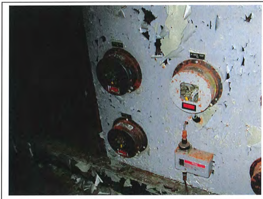
Photo 13: Mercury switches in the Compressor Room of the Engine Room. (September 12, 2014)
